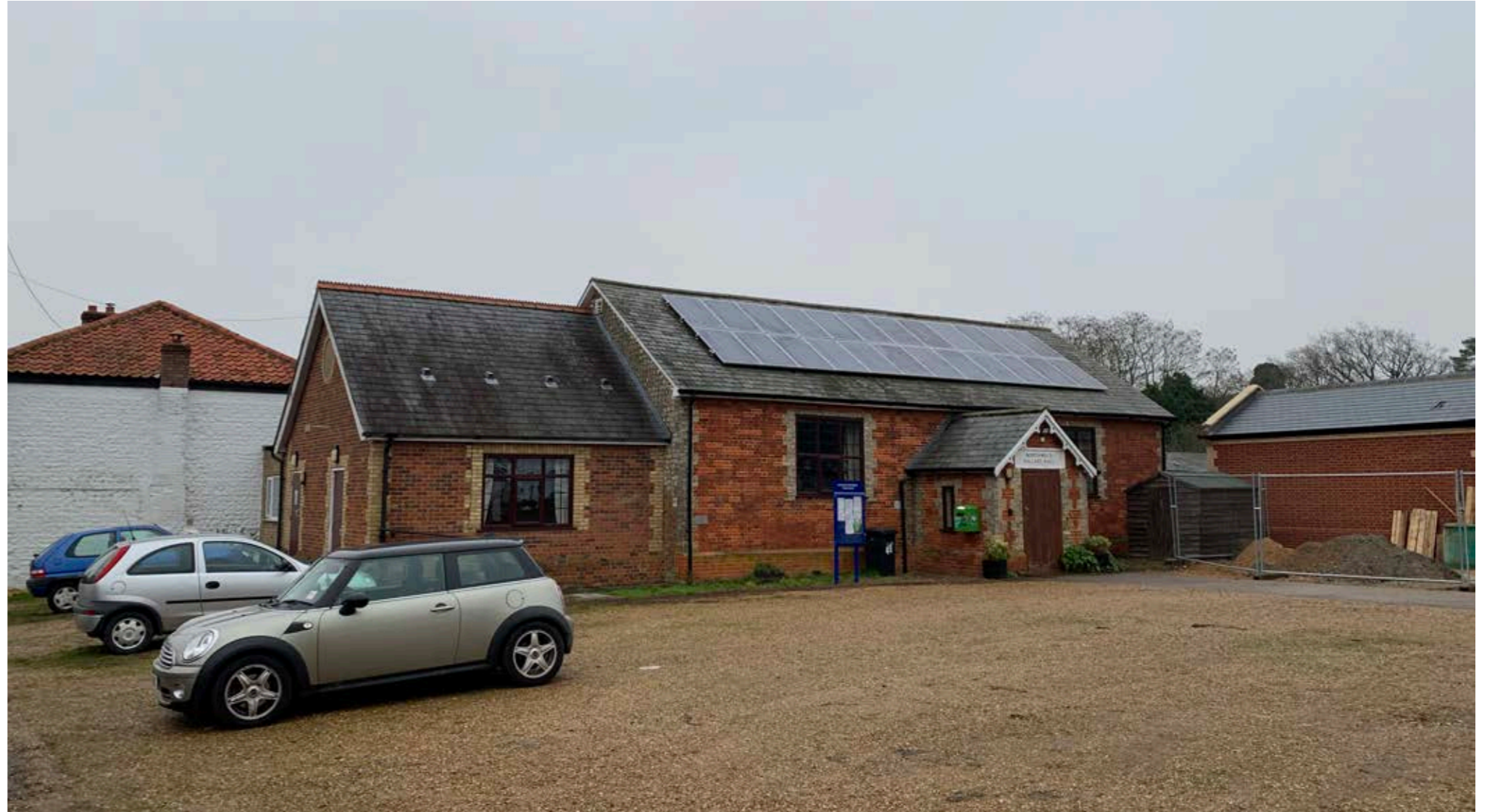
Photovoltaic panel precedent: Northwold Village Hall
