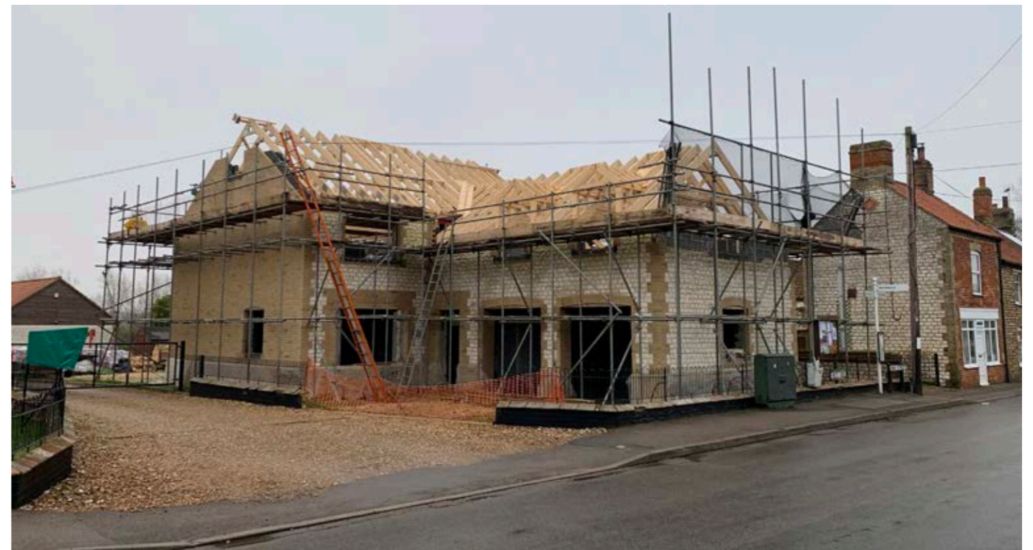
New construction on the High Street
