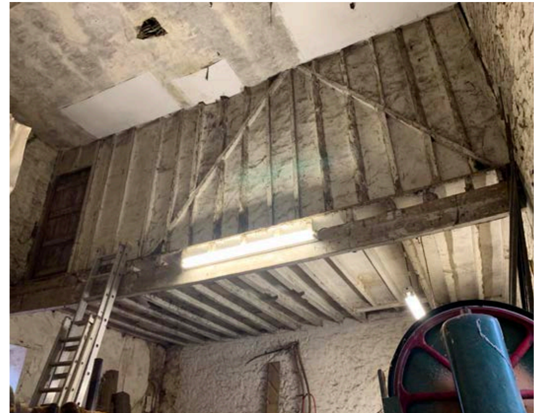
East room with hayloft
