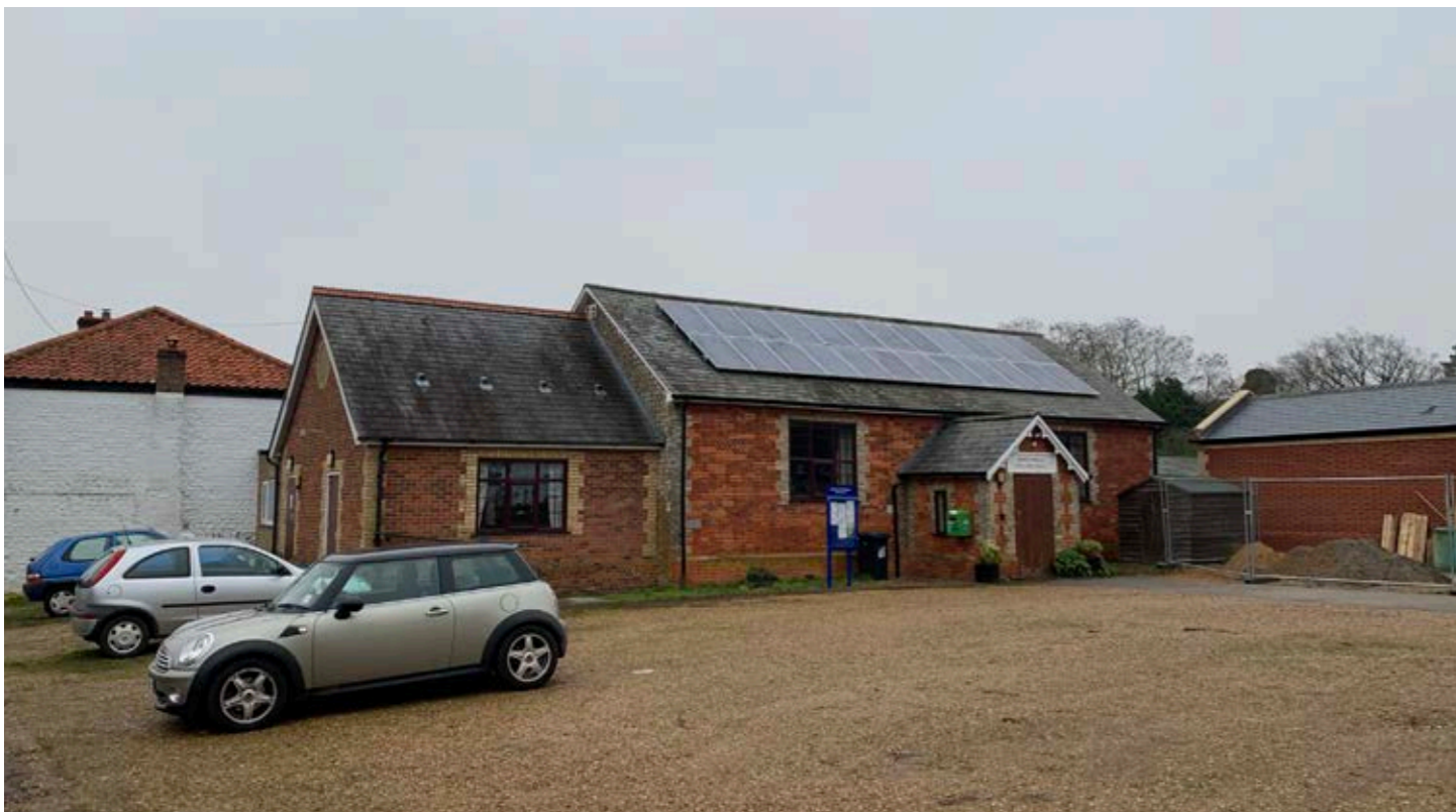
View of Northwold Village Hall
