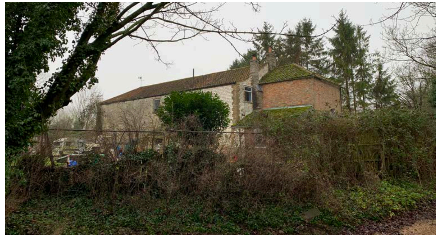
View looking South-East from Common Drove ford crossing
