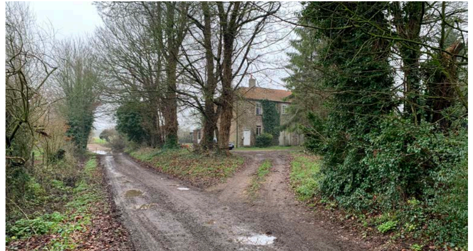
Approach to The Stables from Common Drove
