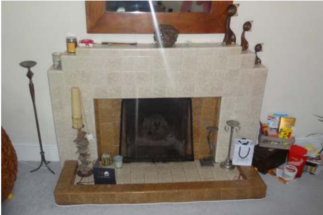
Photograph showing the existing lounge fireplace
