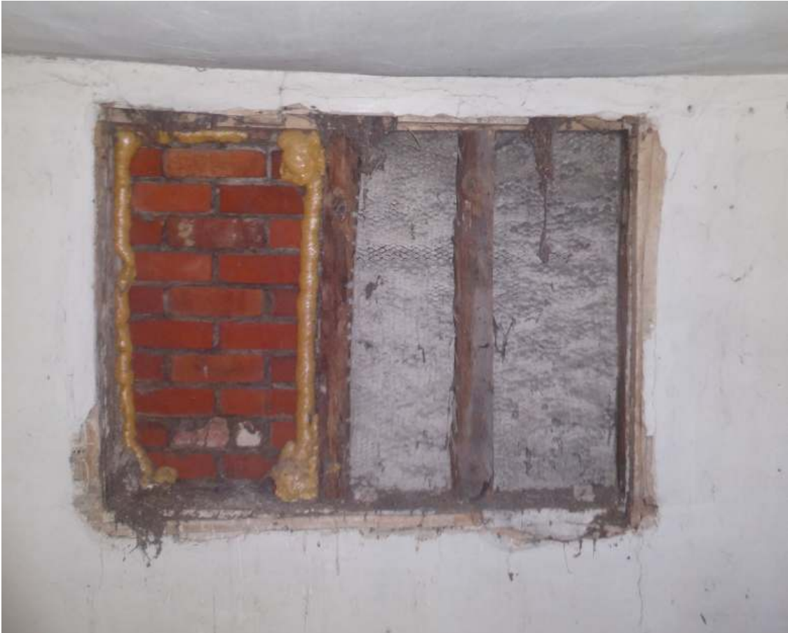
Photograph showing the Existing blocked up rear 2 ND floor window.
