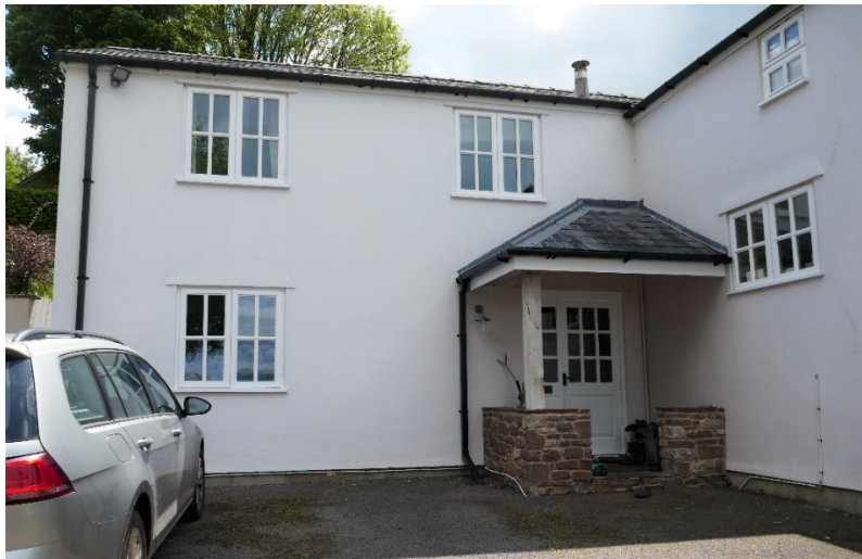
1. The existing porch
