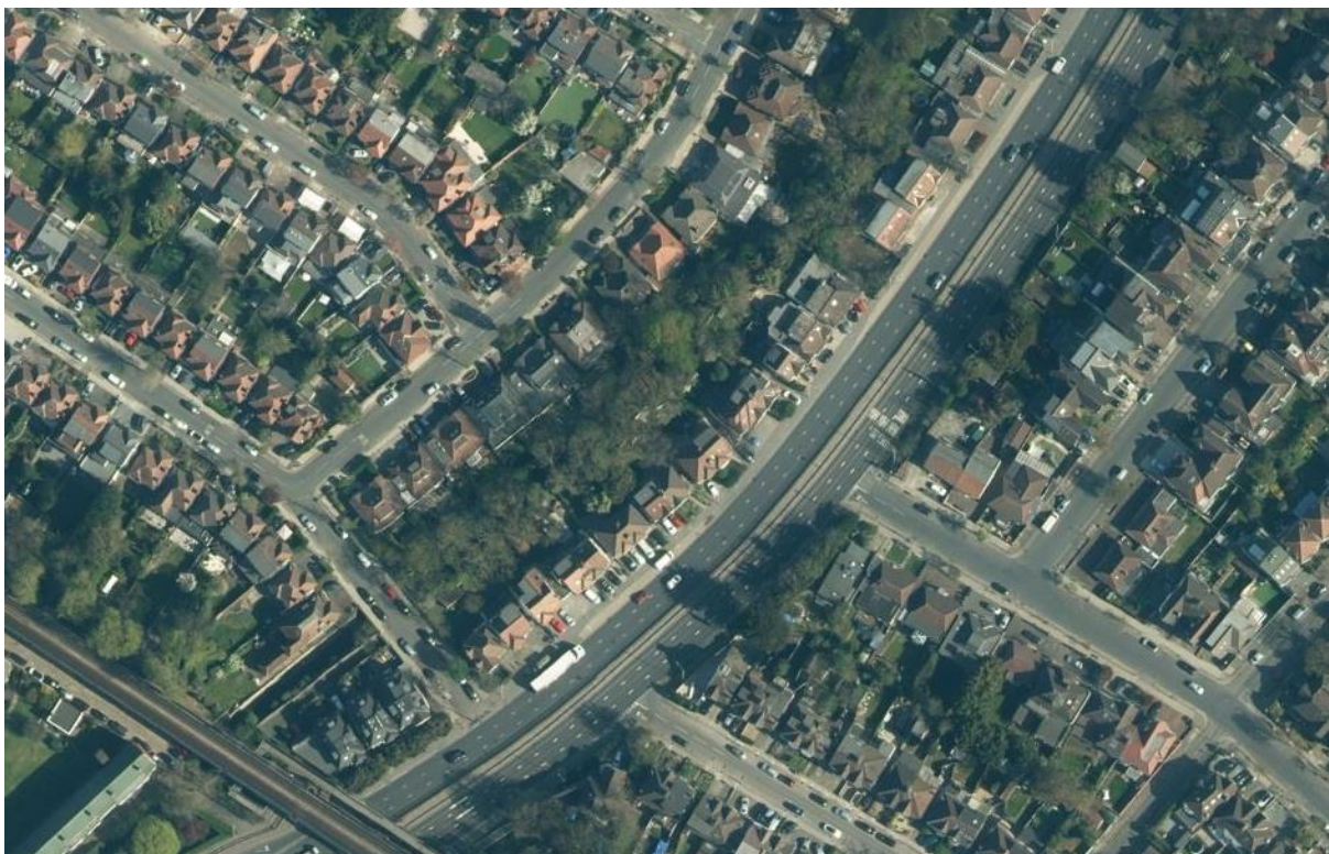
Figure 3 – aerial photograph of the development site.
