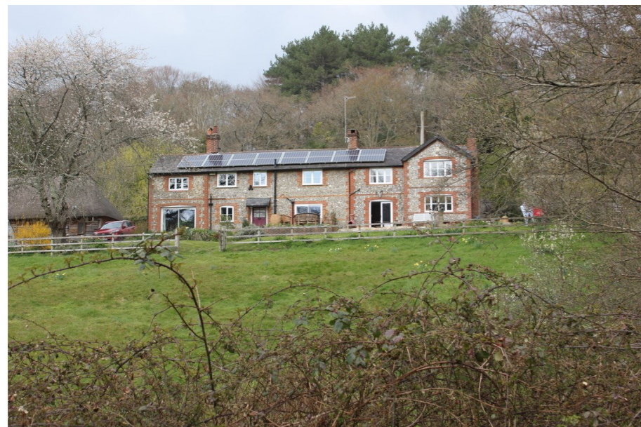
Fig 13. View northwards of Flintstones (Local Building of Interest) from the Avon tributary along the valley floor— houses have been orientated longitudinally on the hillside along the contour line, and fenestrated to take advantage of the south facing views afforded by the elevated position. (Source: SGA April 2021)
