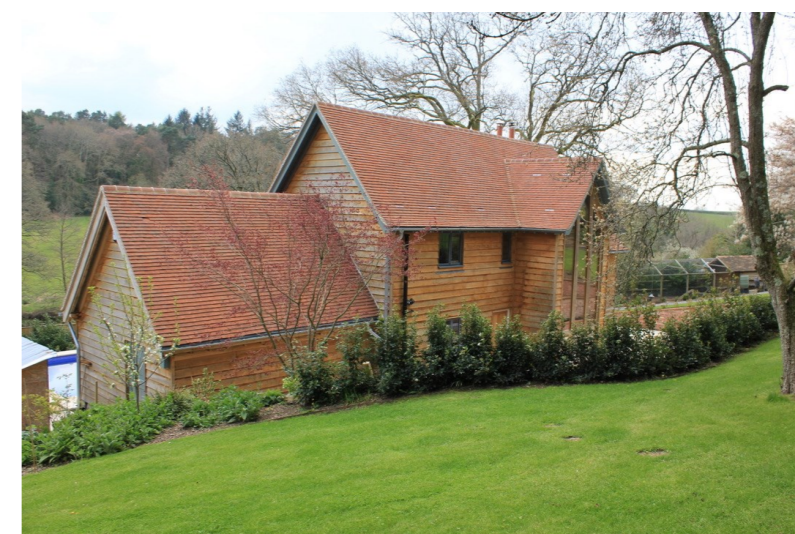
Fig 1. The dwelling viewed from the northeast (front elevation)
