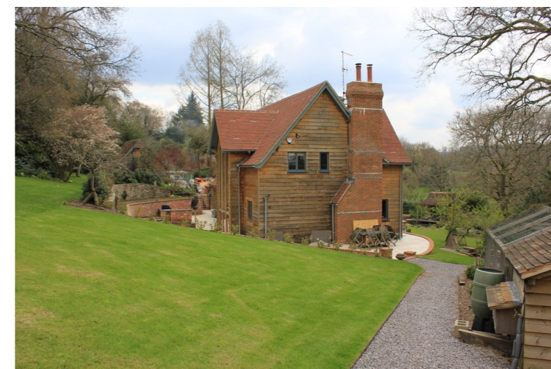
Fig 2. The dwelling viewed from the northwest (Source: SGA April 2021)
