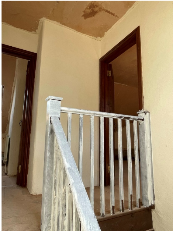
First floor landing
