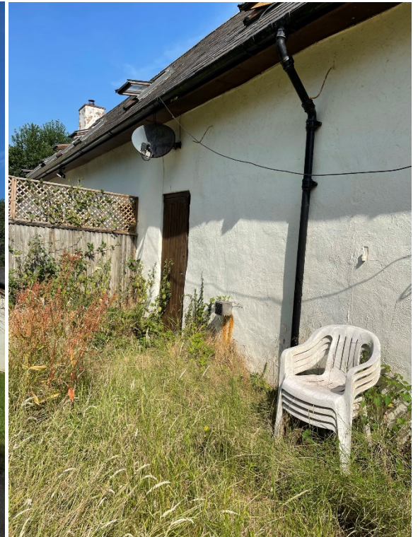
Rear wall with vents & satellite dish
