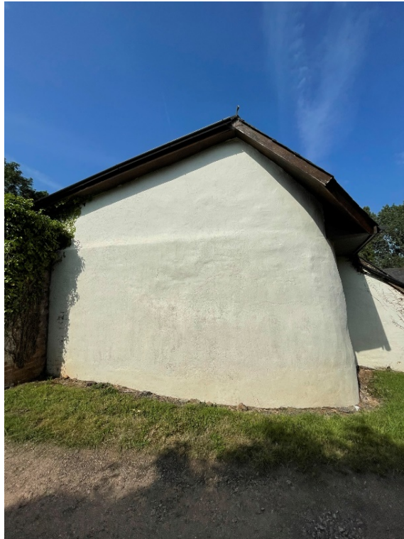
End wall to east
