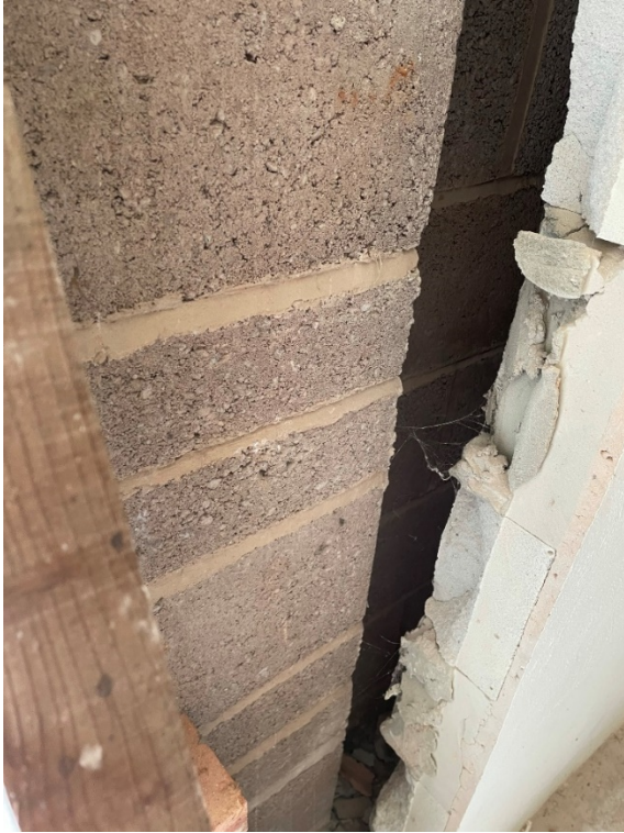
Rear wall - existing blockwork
