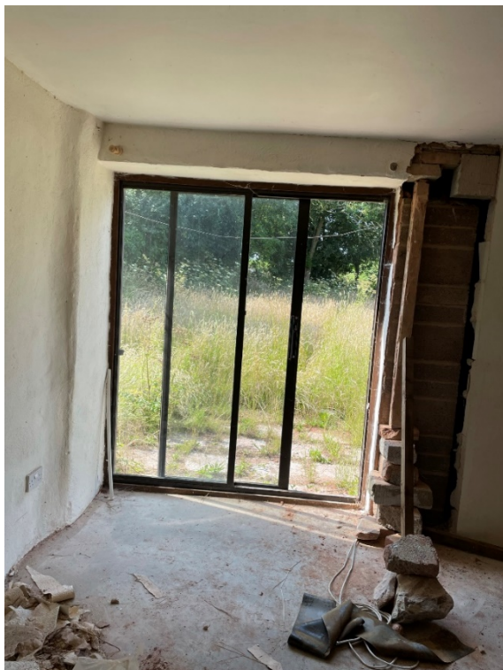
Rear sliding patio doors
