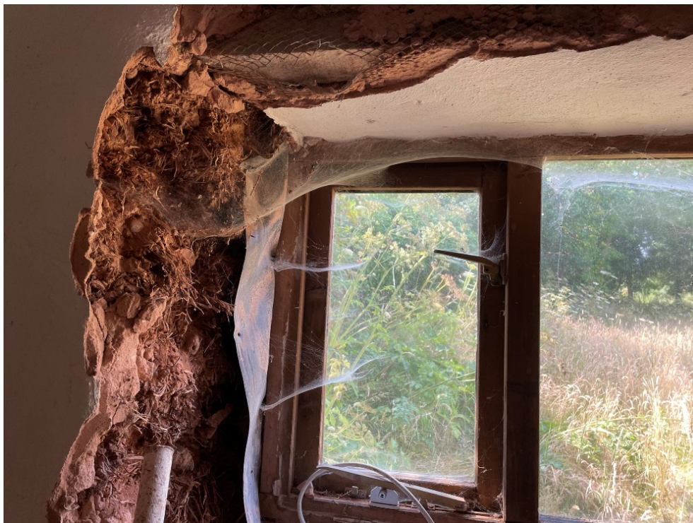
Kitchen window surround showing existing concrete lintel
