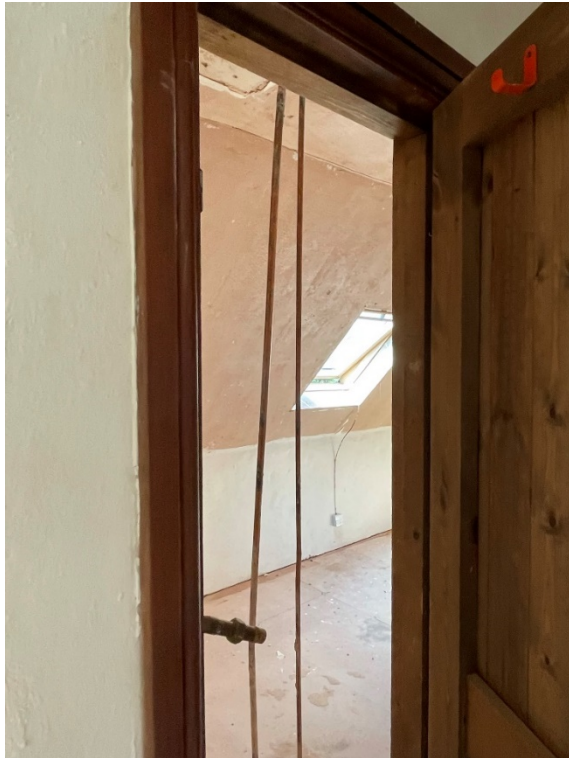
Corridor boiler cupboard removed
