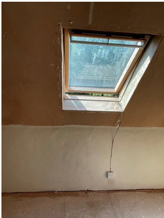
Bedroom 3 – existing rooflight
