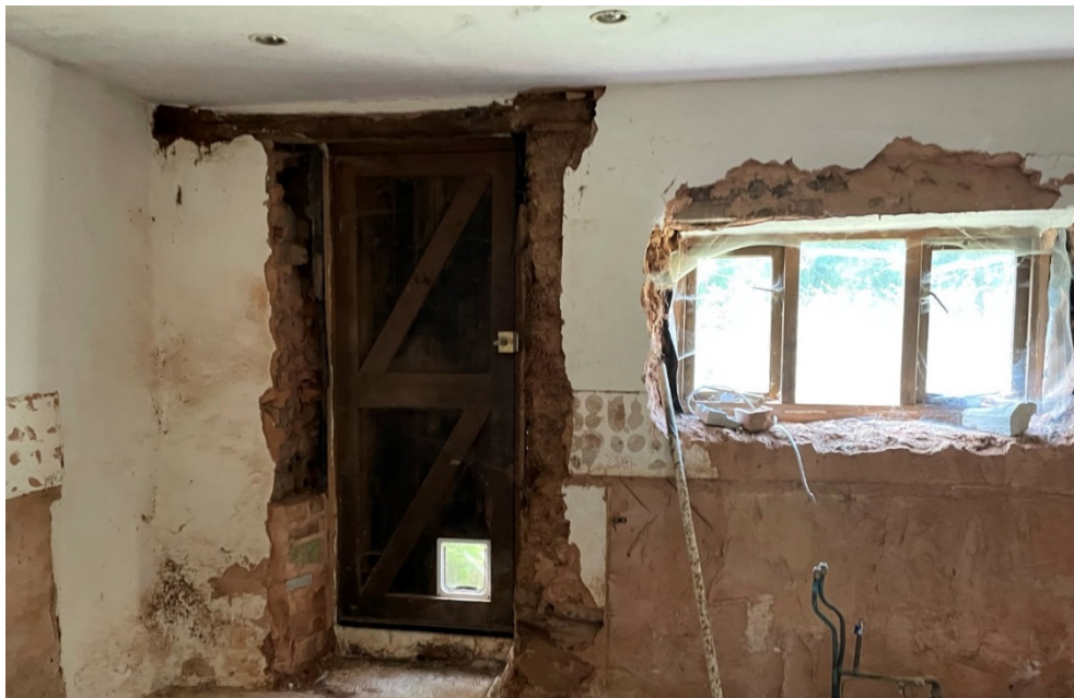
Internal view of kitchen door and window to rear
