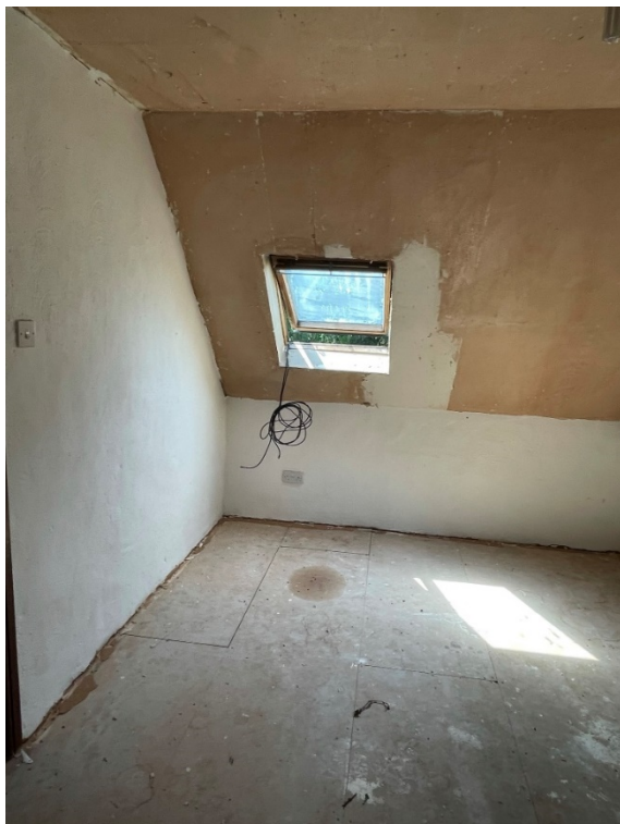
Bedroom 2 – existing rooflight
