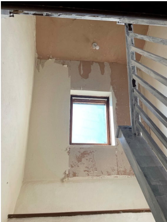
Stairwell roof light as existing
