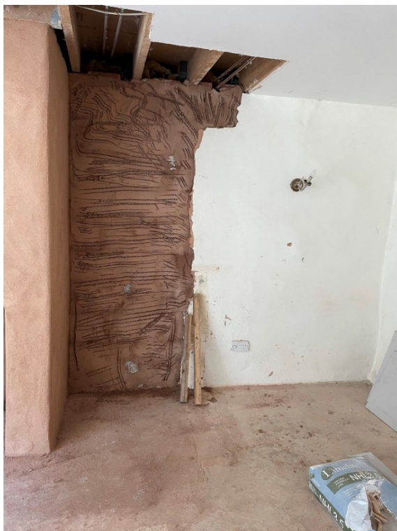
Blockwork / false chimney breast wall removed
