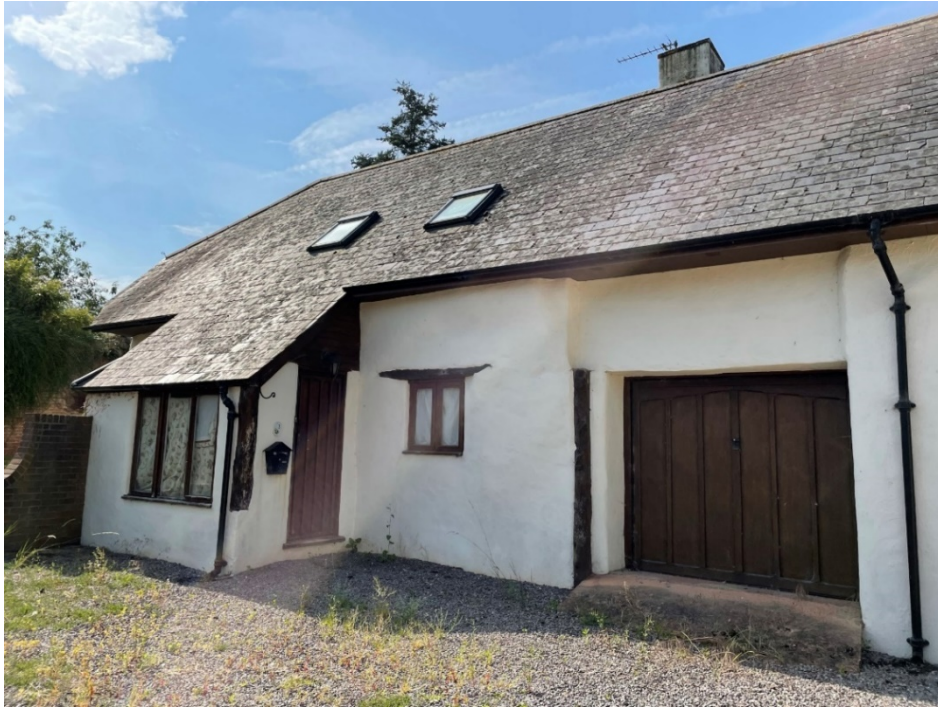
Front entrance to north
