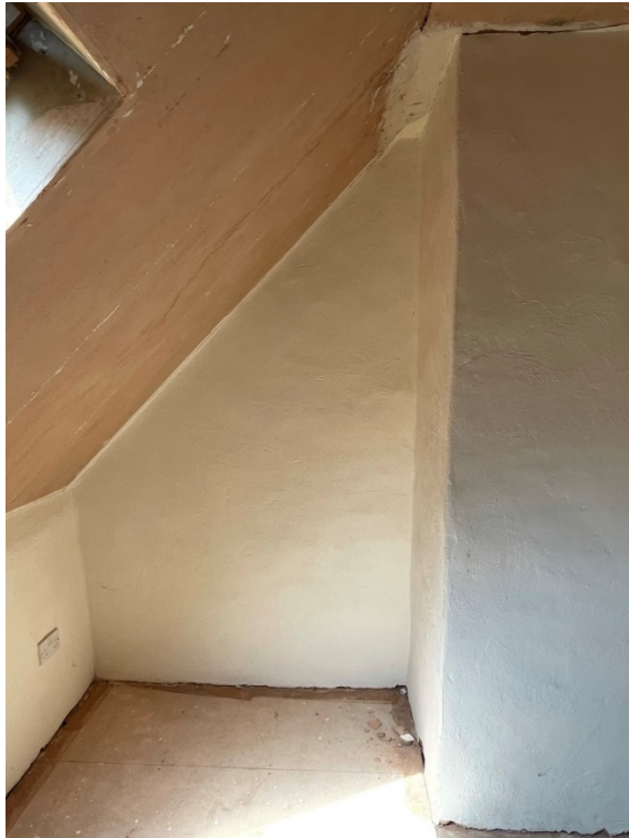
Bedroom 3 – showing existing chimney flue
