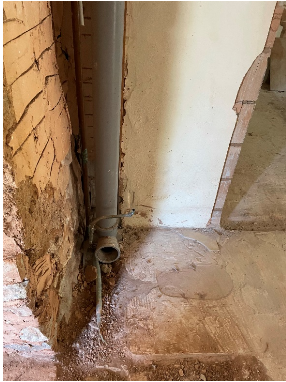
Existing wall & pipework at entrance
