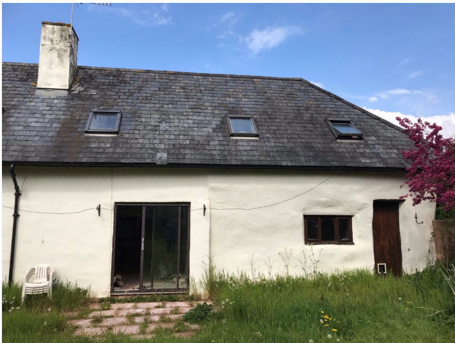
Rear elevation to south
