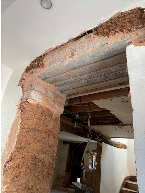
Entrance opening with concrete lintel above
