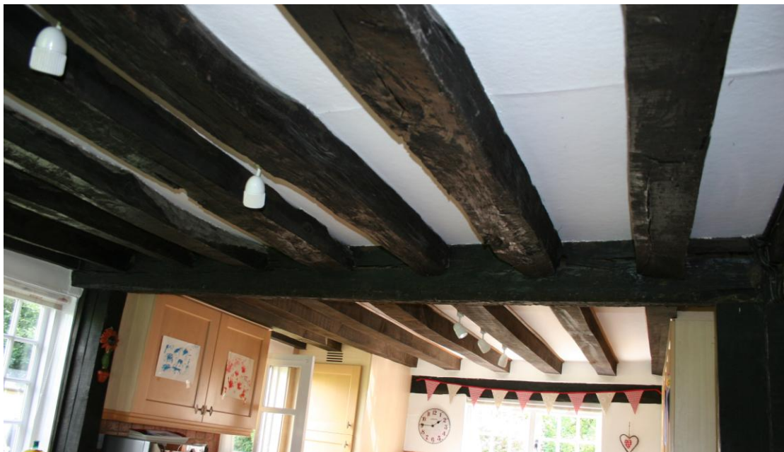
Looking S in the cross-wing Kitchen.
