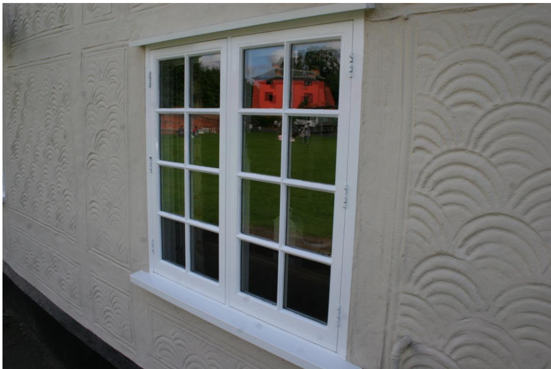
Detail of the replacement windows on the north elevation.
