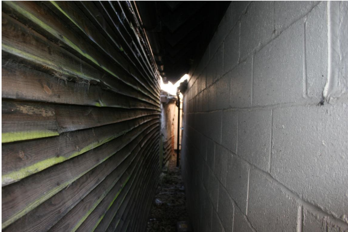
The western wall of the extension alongside the weather-boarded neighbouring building.
