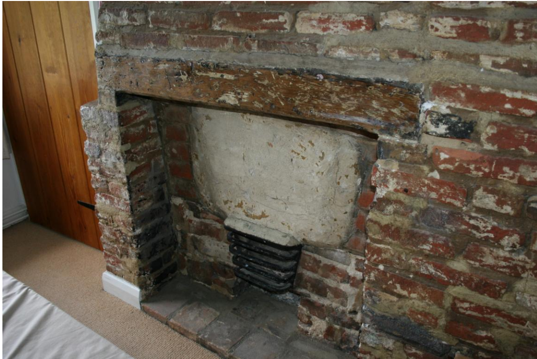
The fireplace in Bedroom 4. Looking E.
