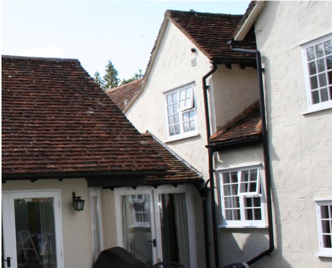
The south elevation gabled extension and stair-tower under a catslide roof.
