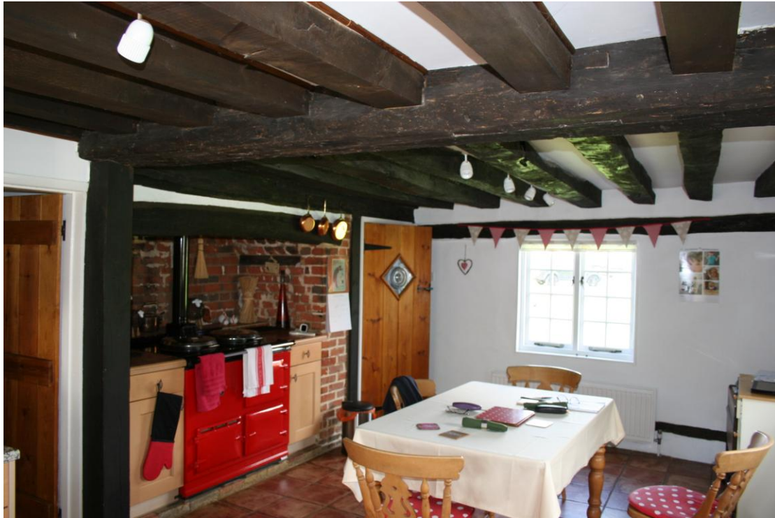
Looking N in the cross-wing Kitchen.
