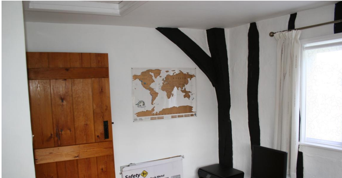
Looking N in Bedroom 3. The spandrel supports a crown post truss.
