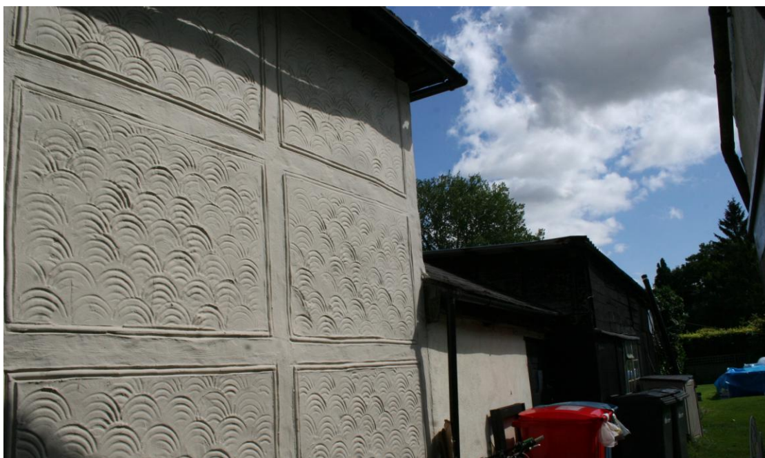
The west elevation with outbuildings in the neighbours ownership.
