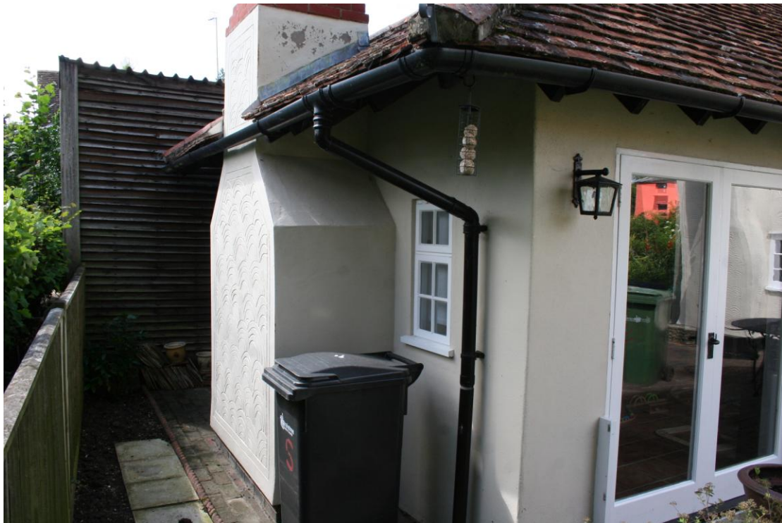
The south elevation of the new extension.
