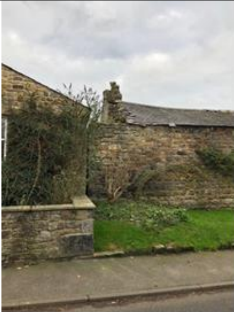
3. Part of gable elevation above the front wall
