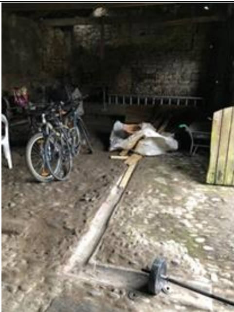
7. Cobble floor with clay drainage channel
