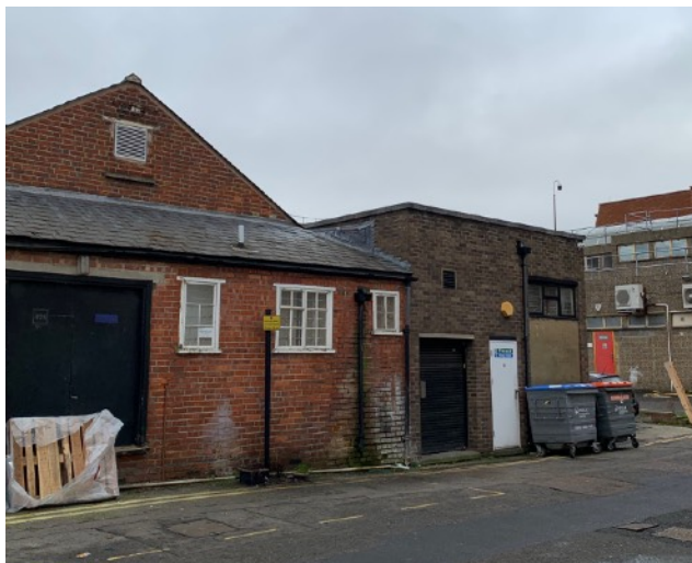
Fig.3 View down Nicholsons Lane to the neighbouring building to the East.
