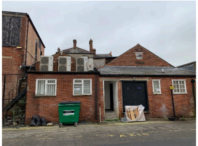
Fig.2 View of the building from Nicholsons Lane.
