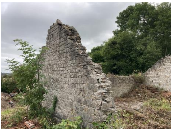
Photo 29: Damaged external wall of Barn 2
