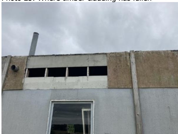
Photo 23: Where timber cladding has fallen
