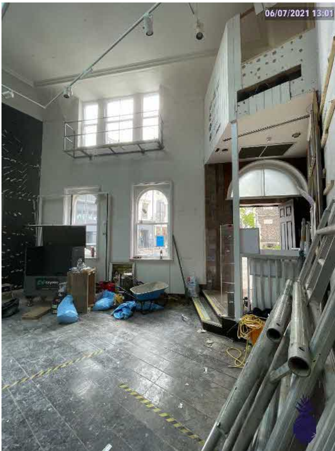
Plate 7: Double-height space when looking towards the main entrance and western elevation.
