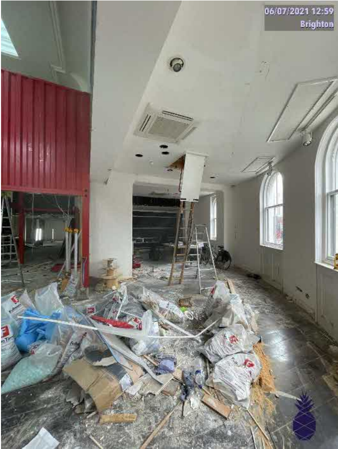
Plate 4: Southern part of the ground floor beneath the mothballed first floor.
