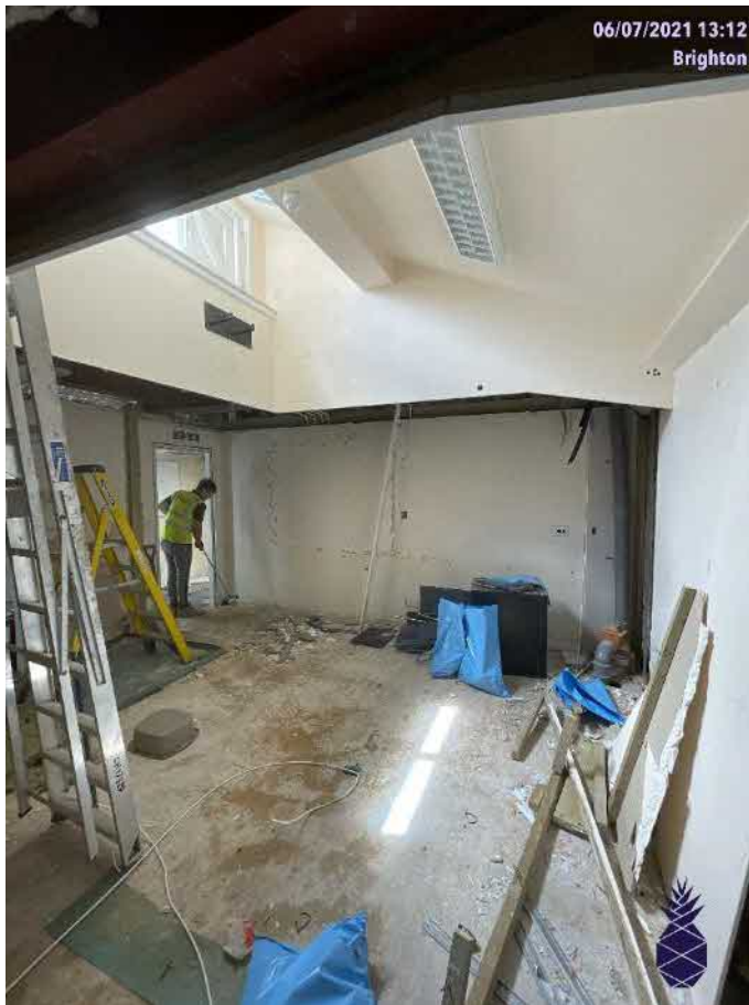
Plate 11: Rear first floor area.
