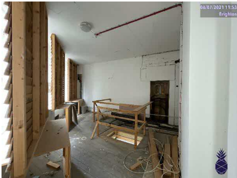
Plate 13: Mothballed first floor only accessible by a hatch.
