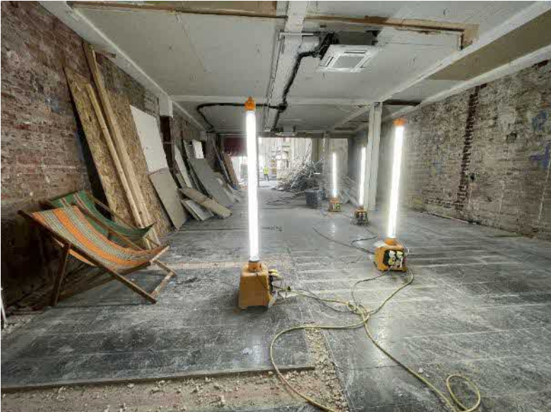
Plate 10: Rear ground floor area.
