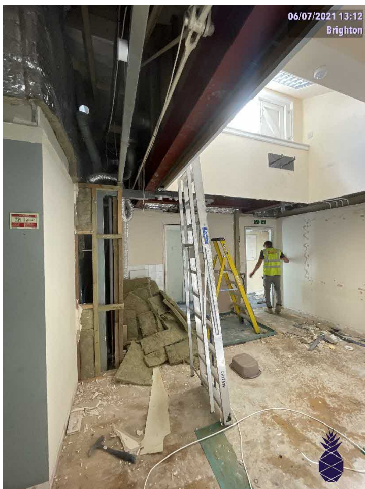
Plate 30: The location of the proposed hoist at first floor level.
