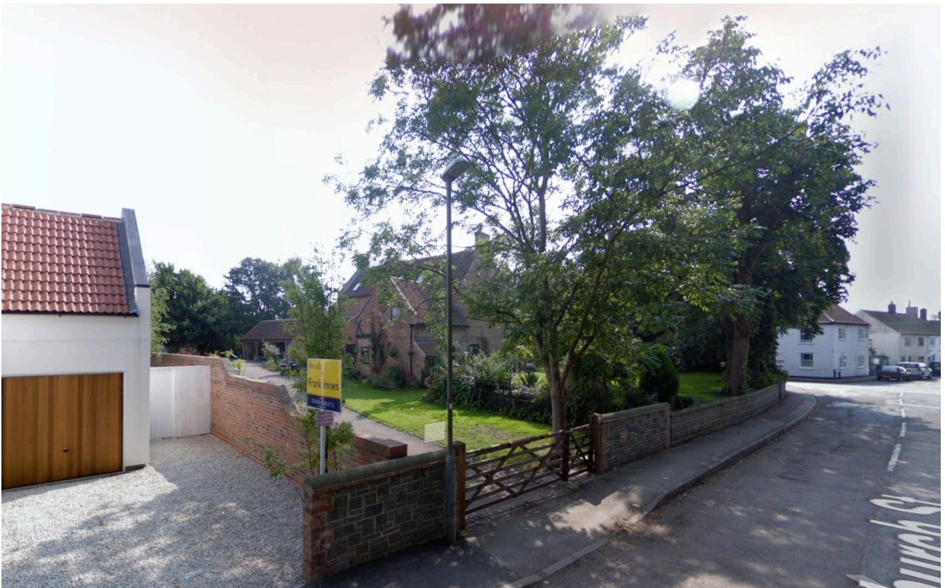
Above: Existing site photograph looking south towards the site showing the partial visibility of the rear (north) elevation.
