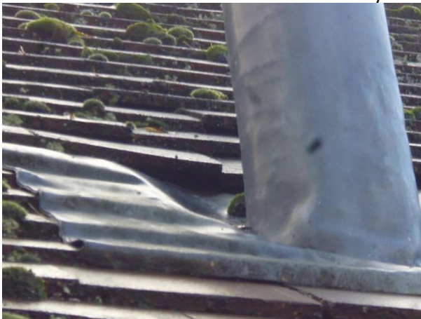
Photo 11: Gaps in Lead Flashing on Chimney
