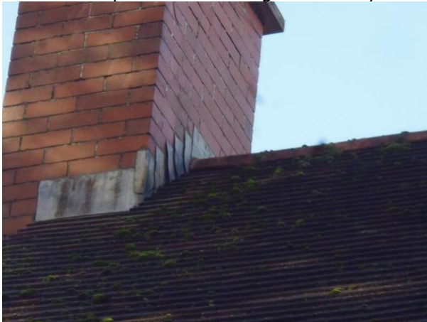
Photo 11: Gaps in Lead Flashing on Chimney
