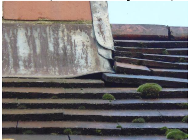
Photo 12: Gap Under Lead Flashing of Chimney
