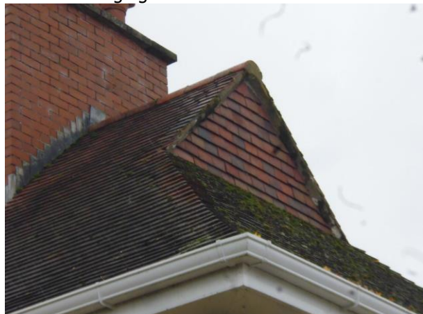
Photo 4: Hanging Tiles on Eastern Elevation
