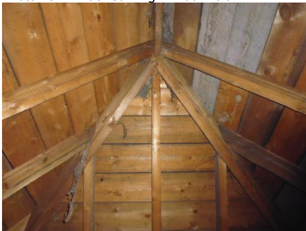
Photo 15: Timber Sarking in Roof Void
