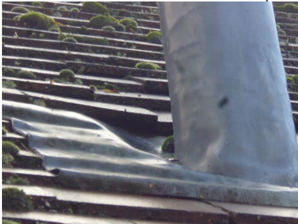
Photo 9: Raised Roof Tile Near Metal Chimney
