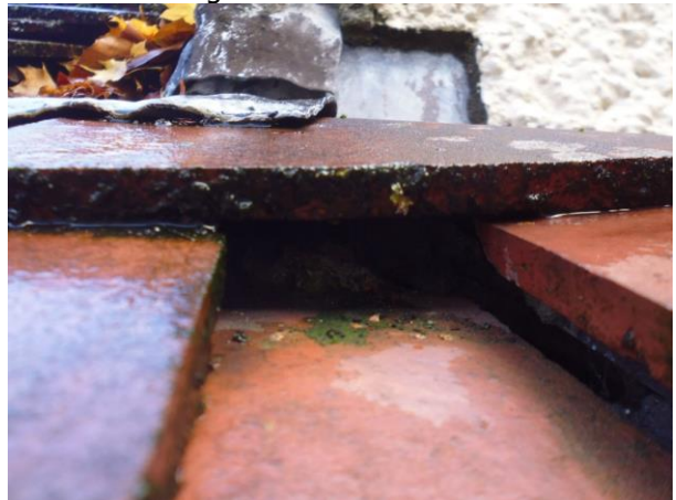
Photo 8: Raised Tile by Chimney
