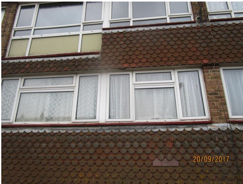
Photo 5 - Tile hanging to front elevation
