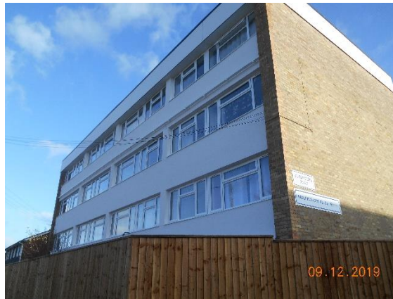
Similar Completed Pilot Block (Prospect Lane)
