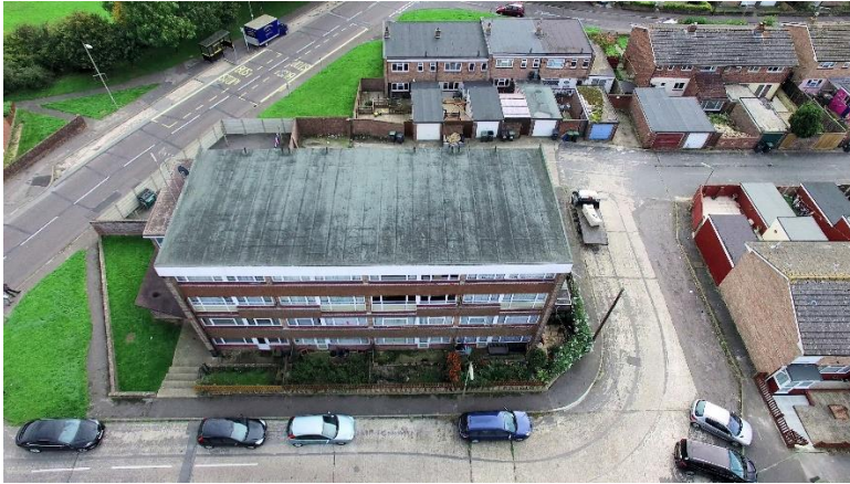
Photo 1 - Arial view of the block (Front Elevation)
