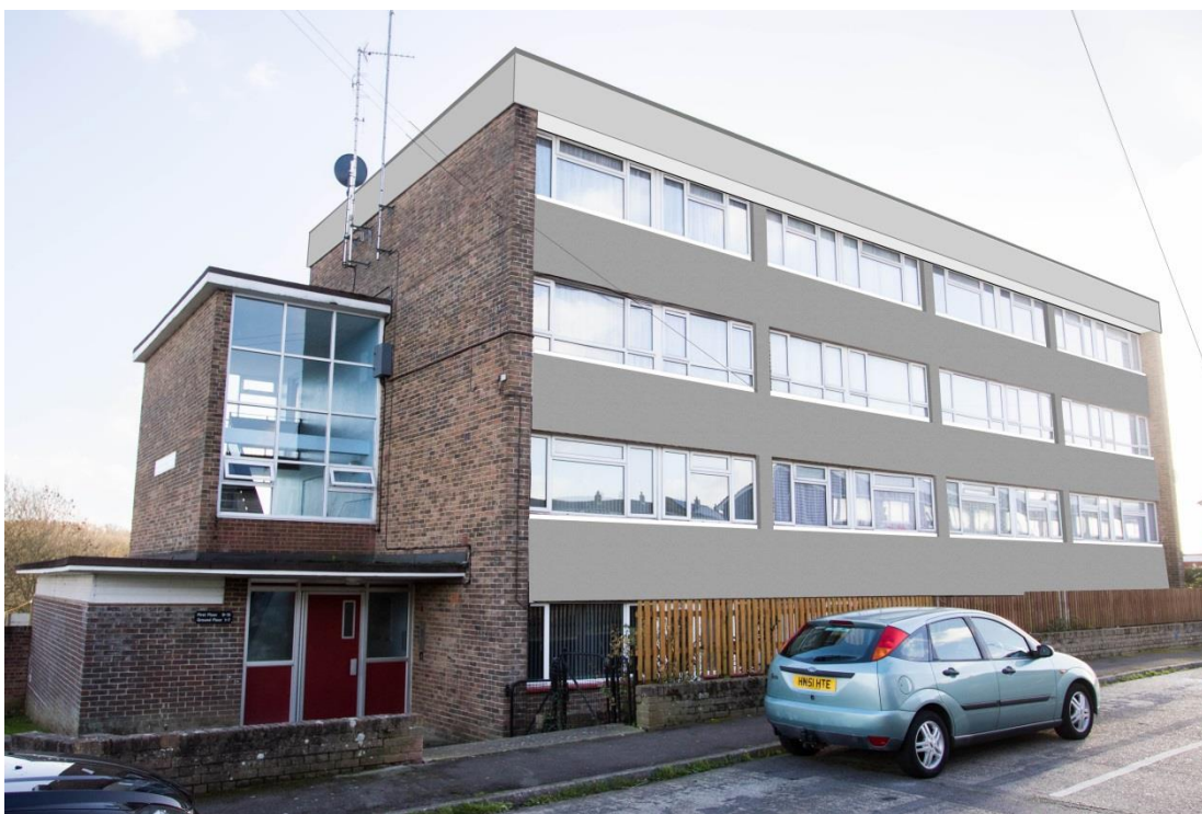
Computer Generated Image showing Render in place of tile hanging. (Note Window design and boundary fencing has not been changed)
