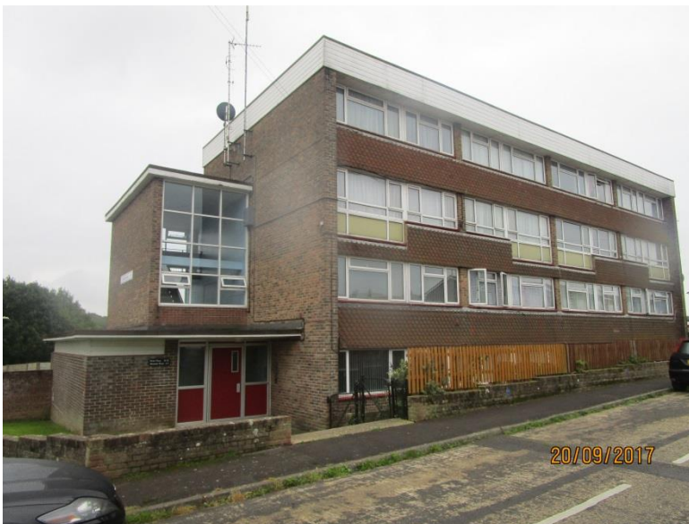
Photo 2 - Front Elevation showing boundary fencing
