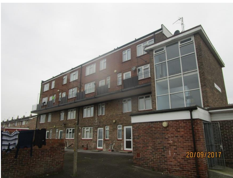
Photo 3 - Rear elevation showing balcony walkway
