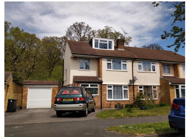
Figure 12: 21 Burnside with a loft conversion dormer.
