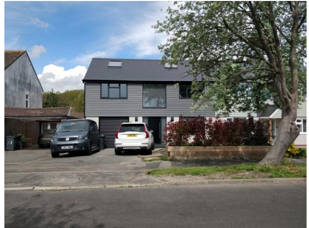
Figure 12: 29 Meadway with a two storey side extension and loft conversion.
