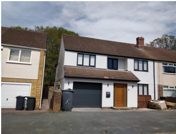
Figure 12: 49 Burnside with a two storey side and rear extension.
