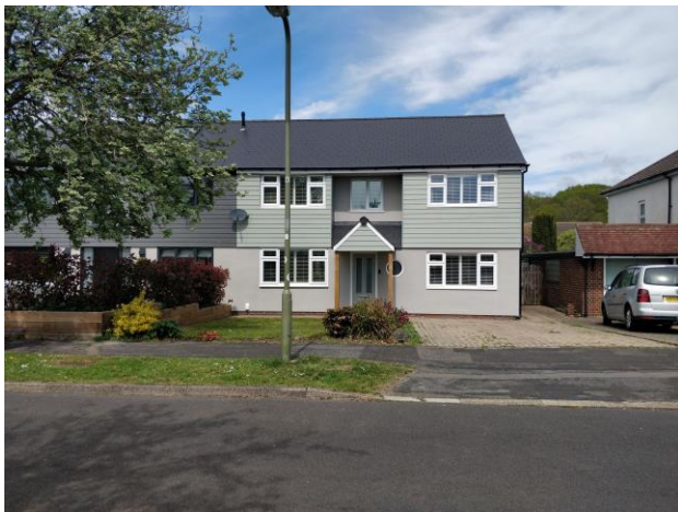
Figure 12: 31 Meadway with a two storey side extension.
