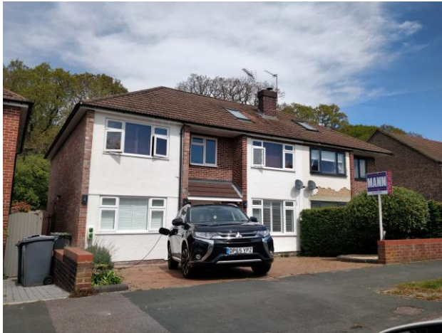
Figure 13: Two storey side and rear extension at 37 Burnside.
