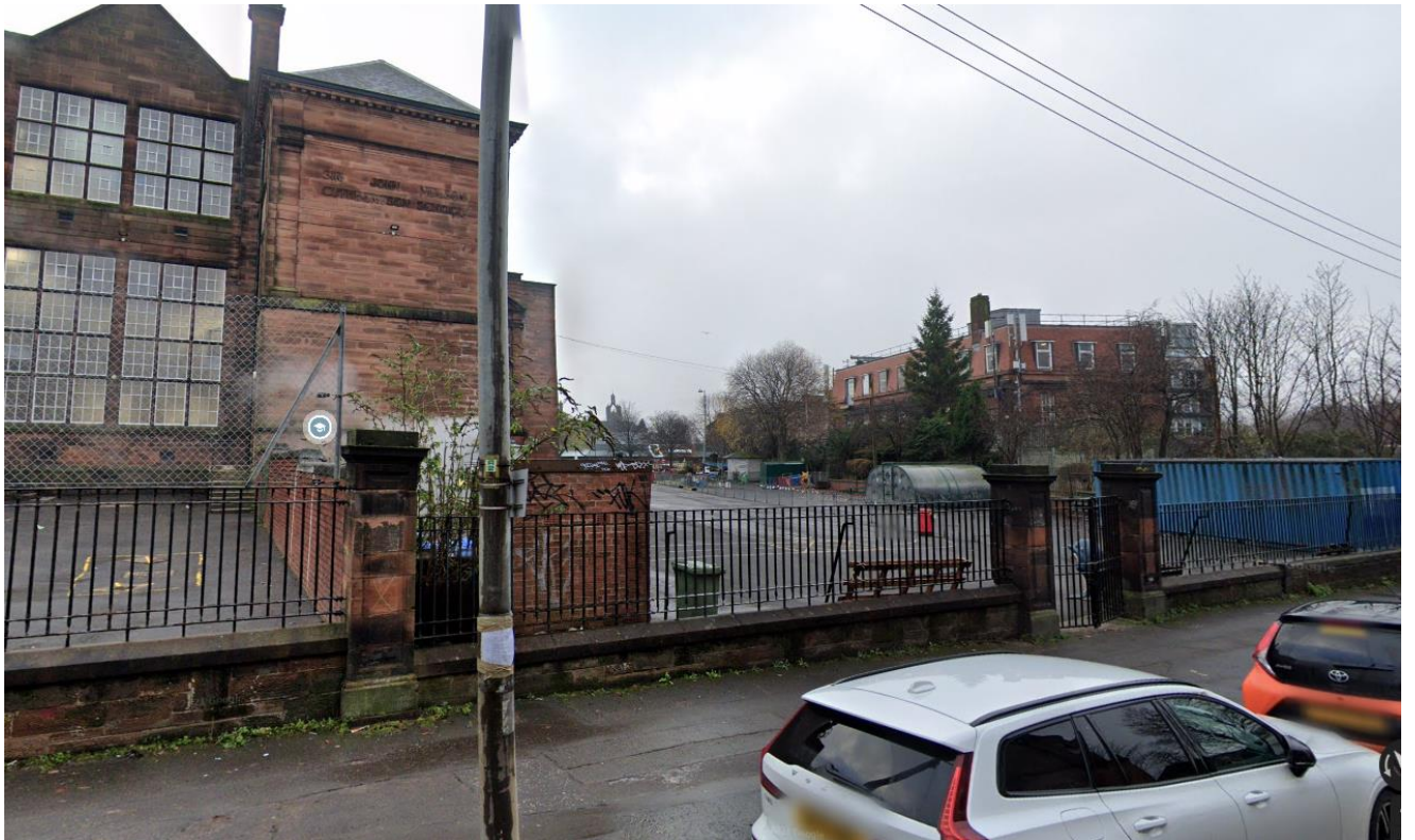
Fig. 2 – Boundary Wall on Coplaw St. of adjacent school building.
