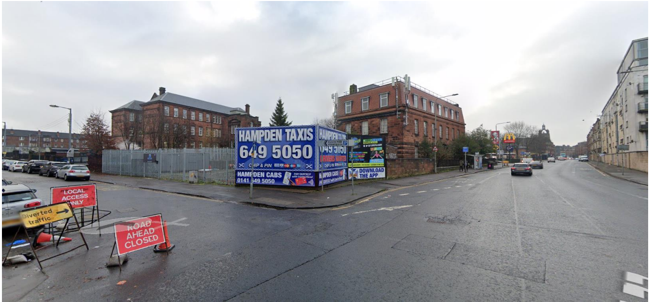
Fig. 3 – Elevation of corner of existing site from Coplaw St. and Pollockshaws junction
