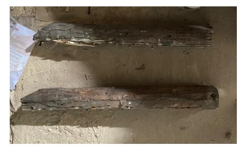
Original ashlaring studs found on site that will be reused when reinstating the rafters.
