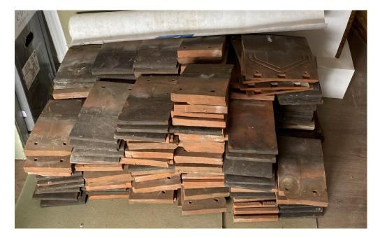
Fortunately the removed roof tiles have been retained on site. They are not original hand made tiles to this rear pitch but a combination of pugmill extruded tiles and machine pressed tiles.
