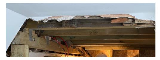
Two of the original vertical studs have been removed. If these are found amongst the materials currently on the ground floor they will be used in the reinstatement of the stud partition.
