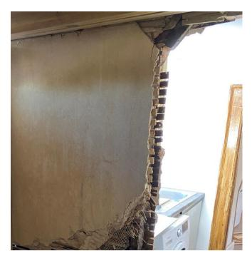
Side of existing dormer showing the lath and render to outside face and lath and plaster to inside face. Doorway in background to front attic room.
