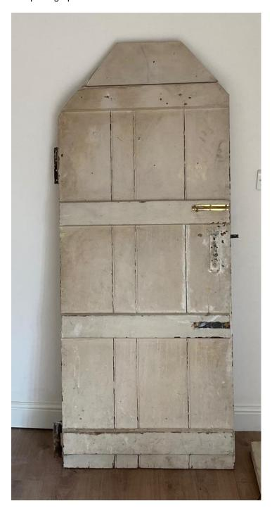
It is a 4 ledged door of random width double Bead and Butt boards with early strap hinges. It appears likely that the two doors upon the second floor may be reused doors that have been altered and adapted for the building. The frames and architraves are more refined than would be expected for these doors.
