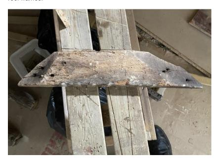
An example of one of the collars that has been removed. Which would appear to have been tosh nailed in place.
