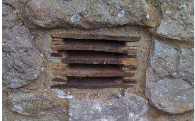
Slate tiles vent in masonry
