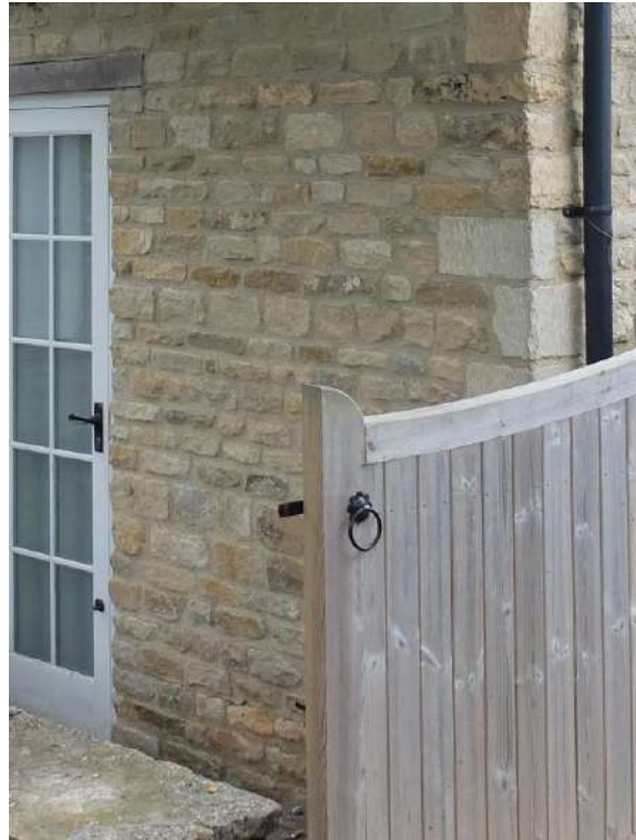
Photos of existing roughly coursed limestone rubble wall of Barley Cottage, proposed to match
