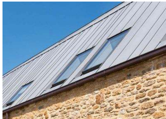
Zinc Quartz standing seam with rooflights
