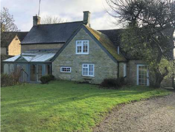
Existing rear elevation of Barley Cottage
