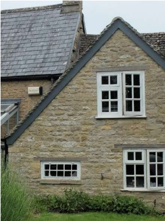
Photos of existing roughly coursed limestone rubble wall of Barley Cottage, proposed to match
