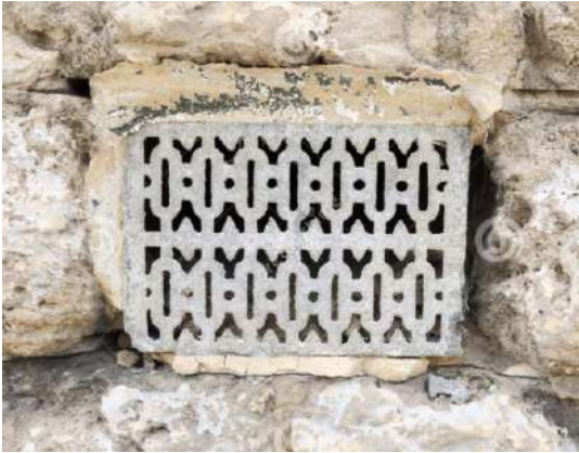
Metal louvered vent in masonry
