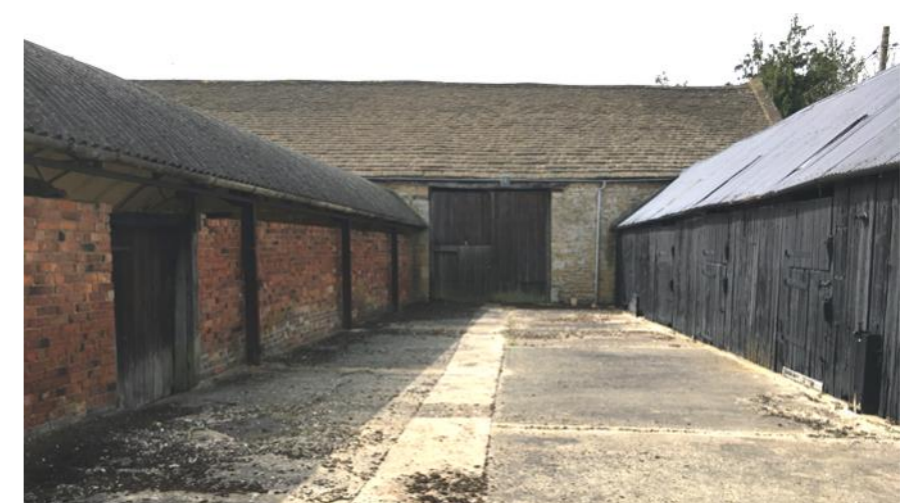
Plate 17: The main barn northern threshing doors, later stables on right and metal roofed shed on left over earlier brick wall occupying footprint of former shelter shed.
