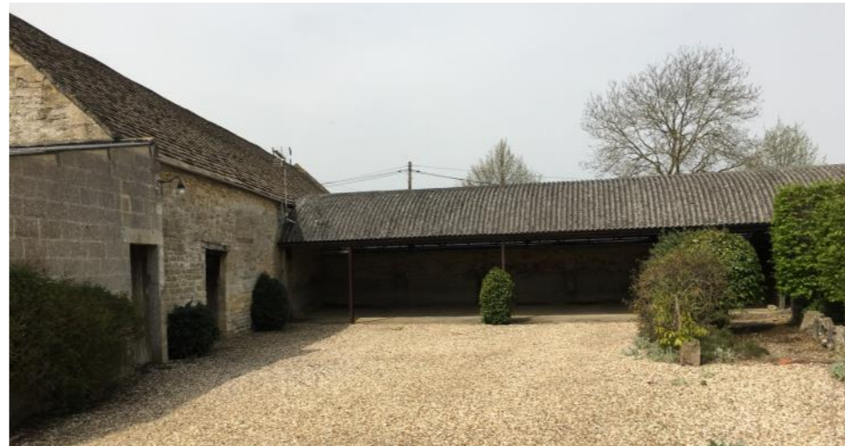
Plate 16: The main barn north elevation of the eastern three bay portion and later concrete block construction, also metal roofed structure behind on footprint of former shelter sheds.
