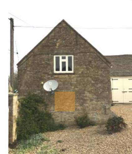
Plate 13: Stable range western gable with position of blocked window shaded.
