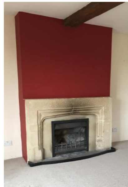
Plate 8-11: (left) Ostensibly early surround but thought to be salvaged and relocated here; (right) Victorian mantel and opening for a range in the extension; (right above) 18th century fireplace with bressumer; (right below) early 20th century brick surround.
