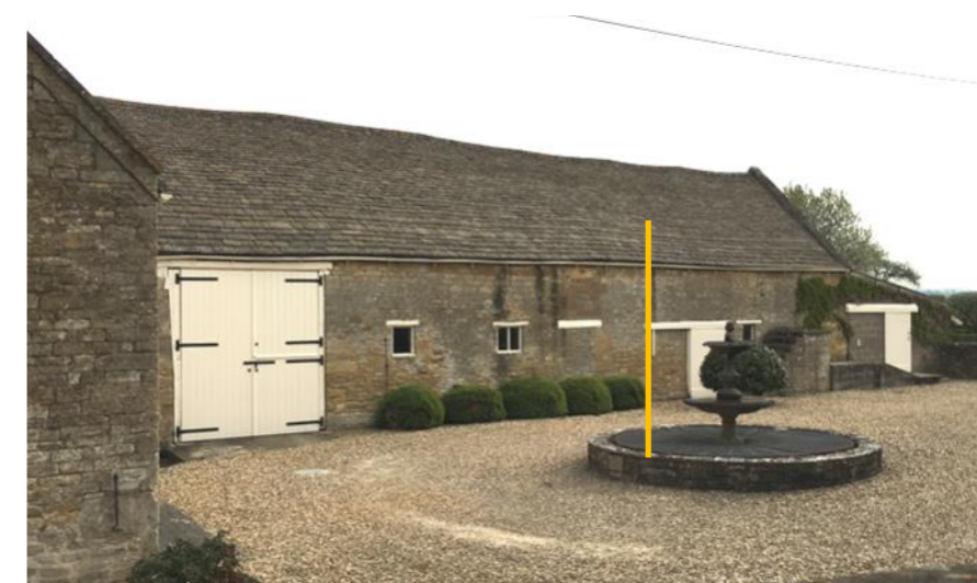
Plate 14: The main barn, the added three bay southern structure is marked with a straight joint just right of the blocked door (marked)
