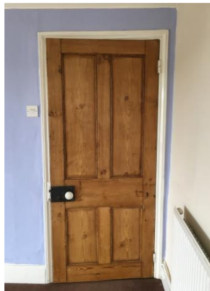
Plate 6-7: (left) Victorian four panel door. (right) typical plank and batten door, of which there are several in the building, with long strap hinges, these with rounded ends.
