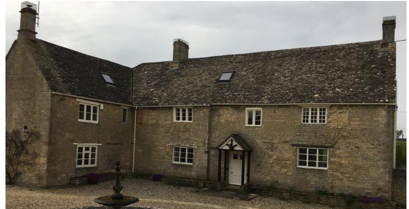
Plate 2-3: Old Foxcote Farm northern yard elevation (above) and extended Victorian range (below). The elevations on all sides of the building show evidence of extension in an easterly direction with the red brick elements being the latest. The single storey red brick structure below features only modern features (doors and skylights and all interiors) and the brickwork also appears less consistent with the two storey section to the right. It may be that this portion was rebuilt or added more recently though we have assessed it as broadly Victorian in overall date based upon the map evidence.
