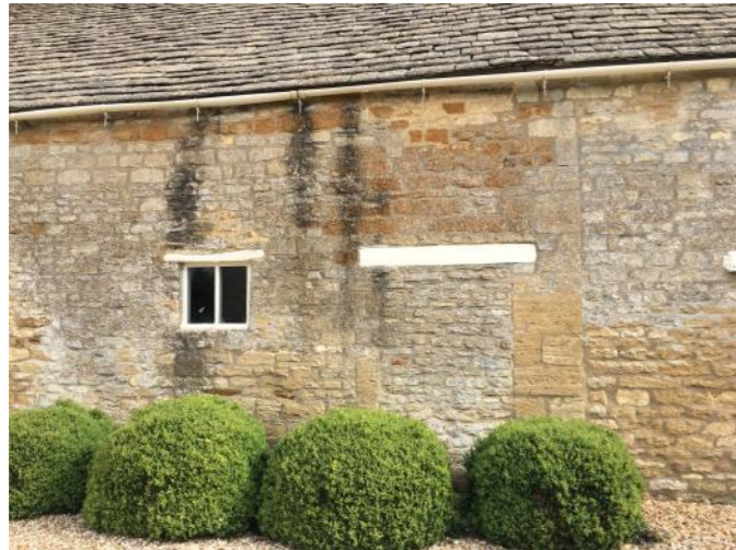
Plate 15: The main barn, blocked door and straight joint showing extension point to east.
