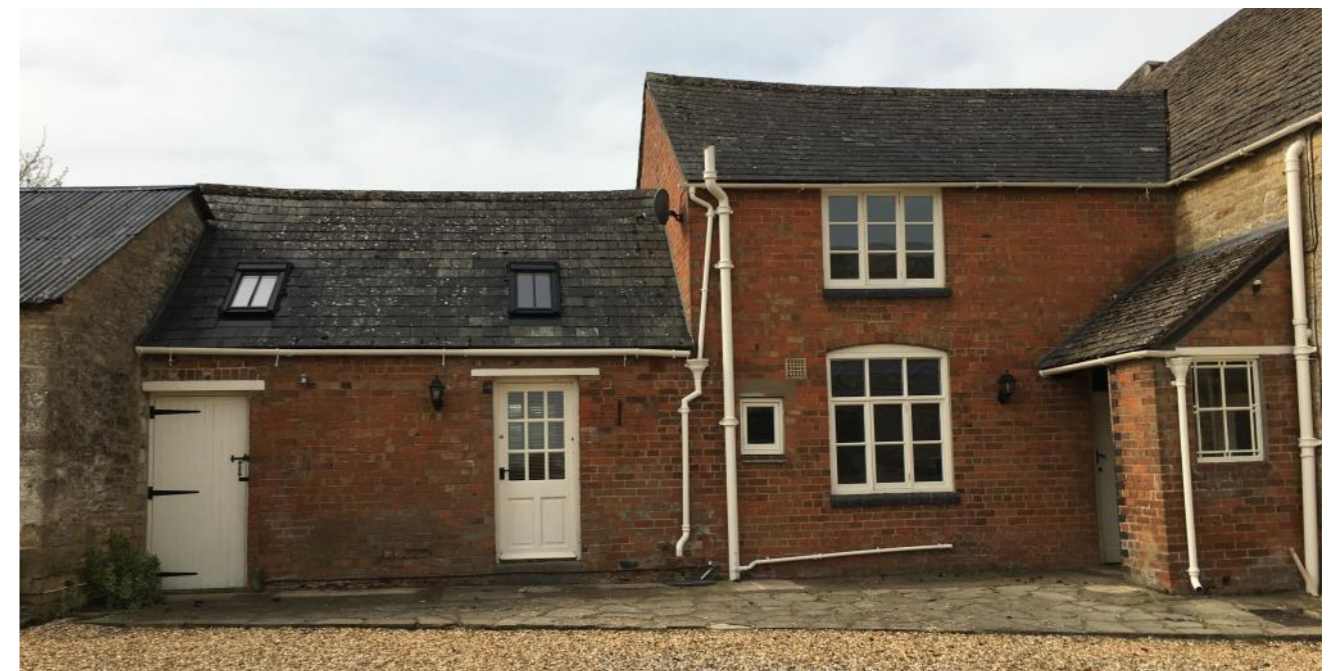
Plate 2-3: Old Foxcote Farm northern yard elevation (above) and extended Victorian range (below). The elevations on all sides of the building show evidence of extension in an easterly direction with the red brick elements being the latest. The single storey red brick structure below features only modern features (doors and skylights and all interiors) and the brickwork also appears less consistent with the two storey section to the right. It may be that this portion was rebuilt or added more recently though we have assessed it as broadly Victorian in overall date based upon the map evidence.
