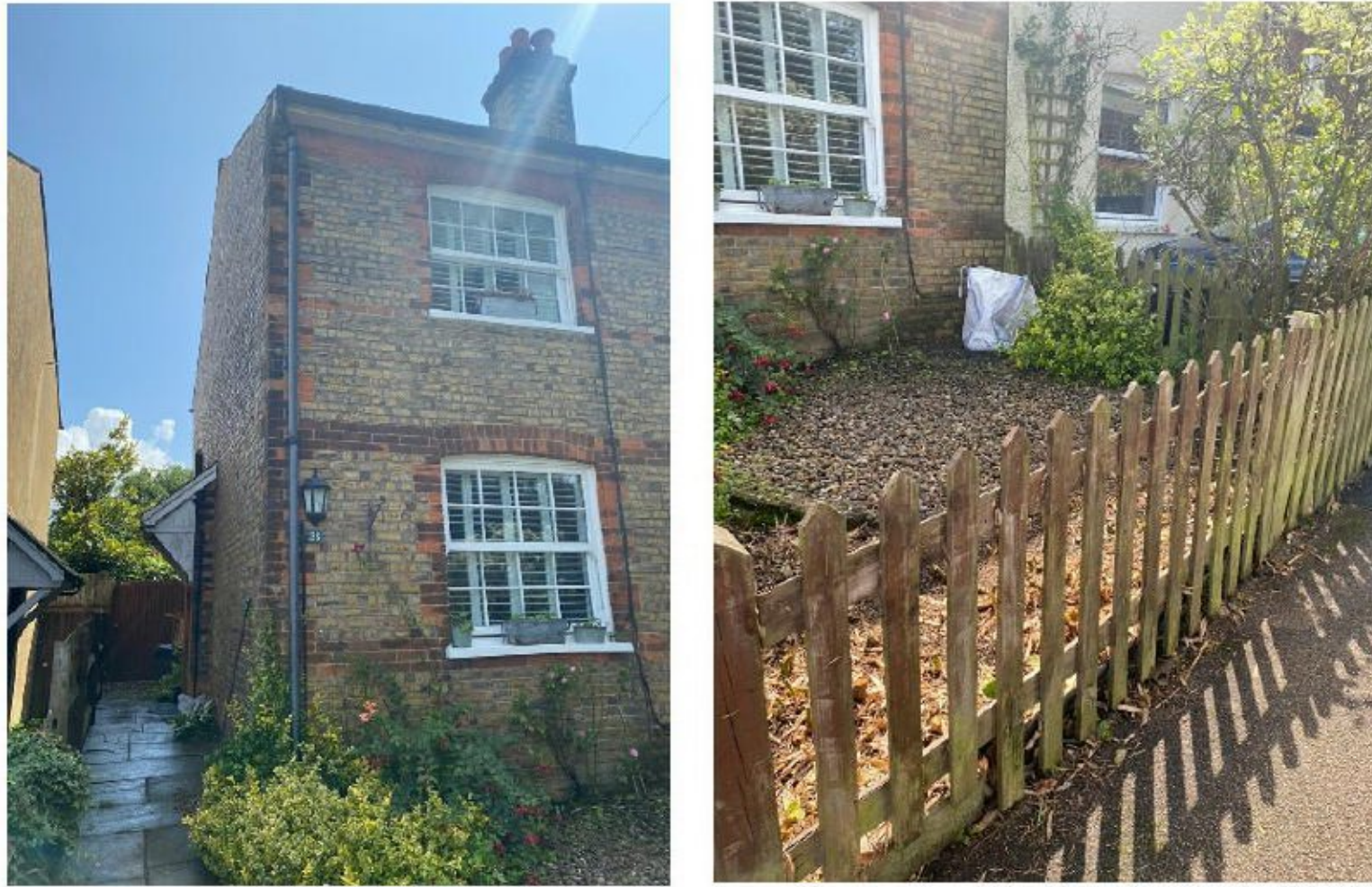
28 Station Road – Front façade and front garden
