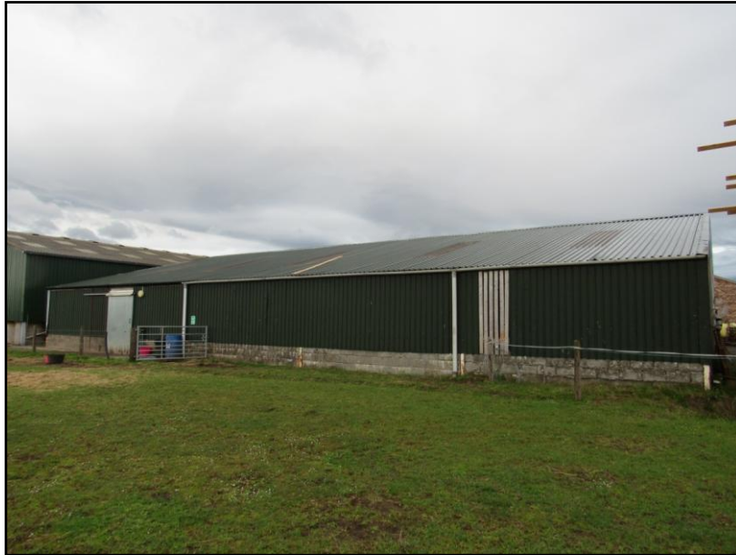
Figure 17. Agricultural shed – western elevation.
