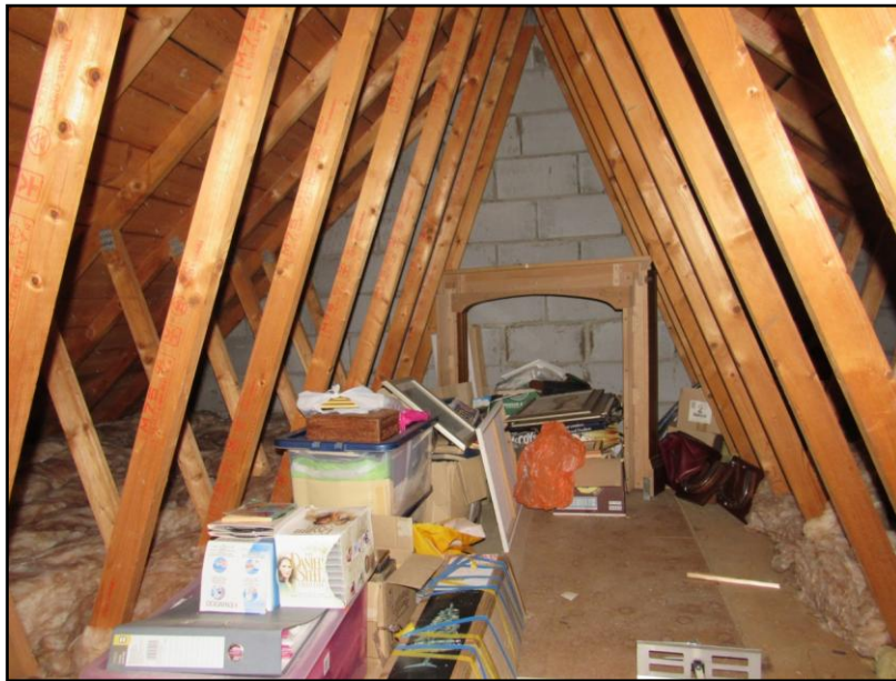
Figure 14. Roof void labelled B in Figure 3.
