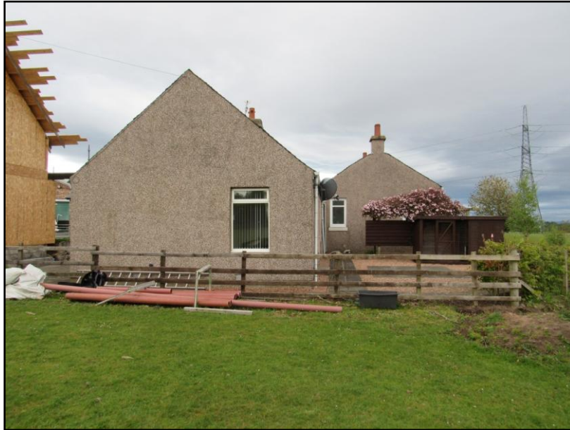
Figure 6. Farm Cottage – western elevation.
