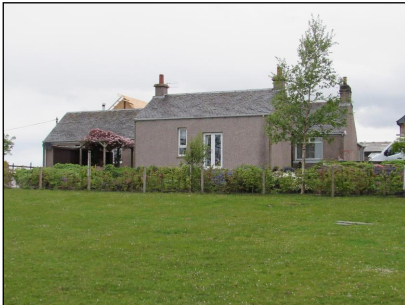
Figure 7. Farm Cottage – southern elevation.
