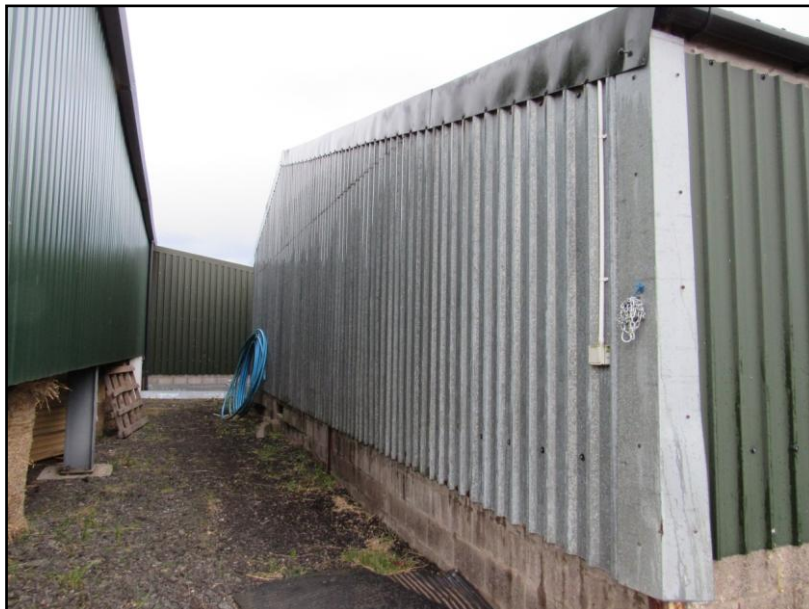
Figure 18. Agricultural shed – northern elevation.
