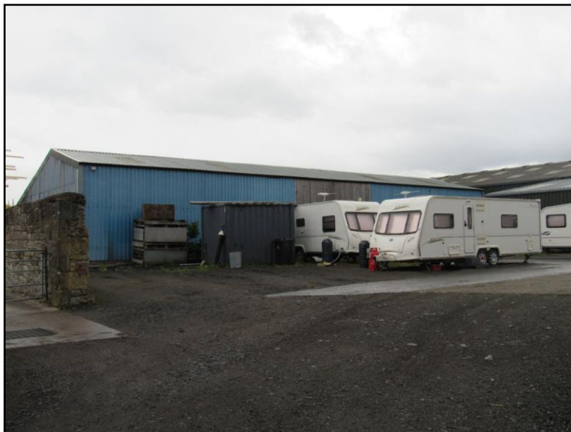
Figure 16. Agricultural shed – eastern elevation.
