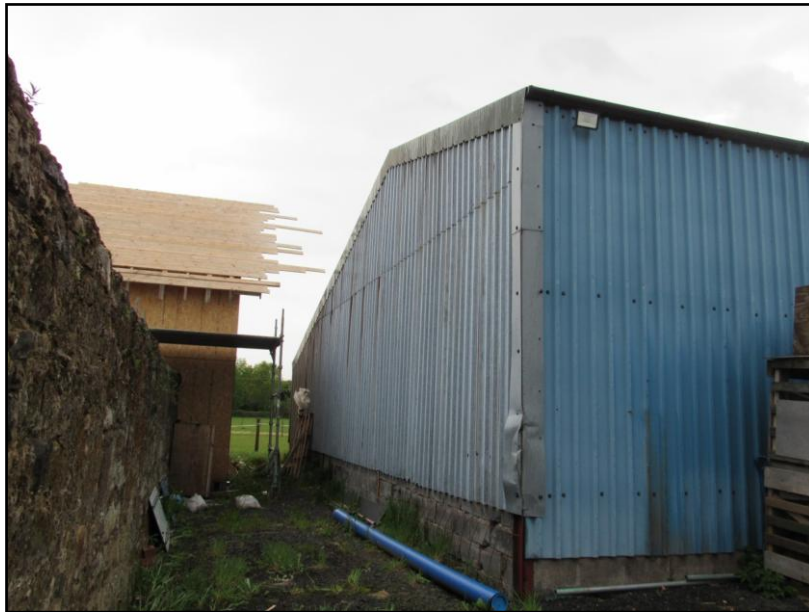
Figure 19. Agricultural shed – southern elevation.
