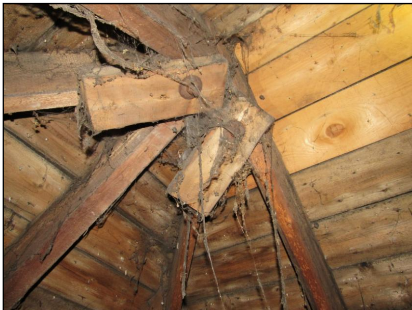
Figure 13. Potential roost sites across the roof are obscured by cobwebs.
