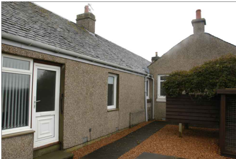
Detail of existing farmhouse
