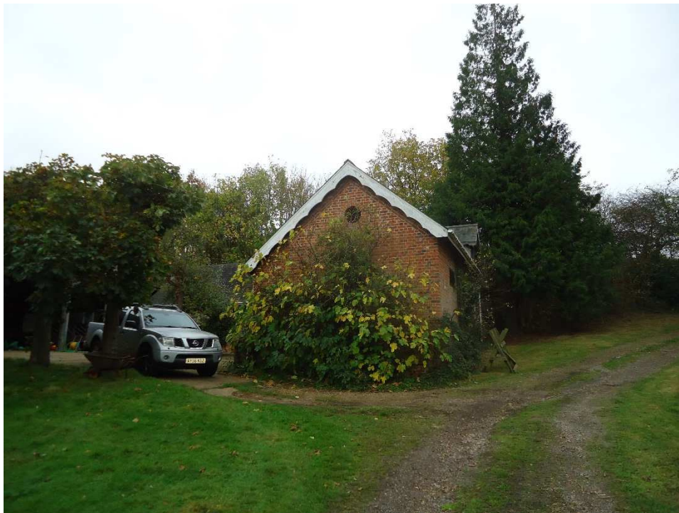
Figure 52: Existing farm buildings.
