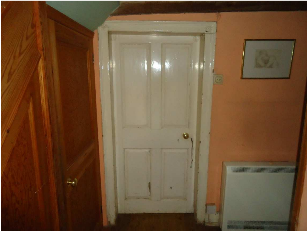
Figure 41: Four panel door leading into brick range from lobby.
