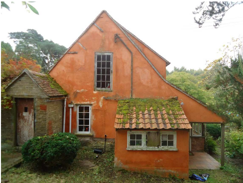
Figure 50: North gable end of the house.
