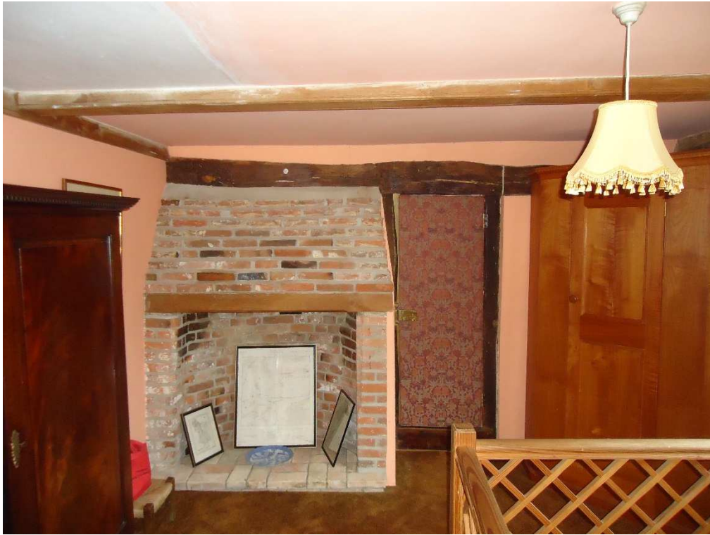
Figure 25: C17 fireplace in parlour chamber.
