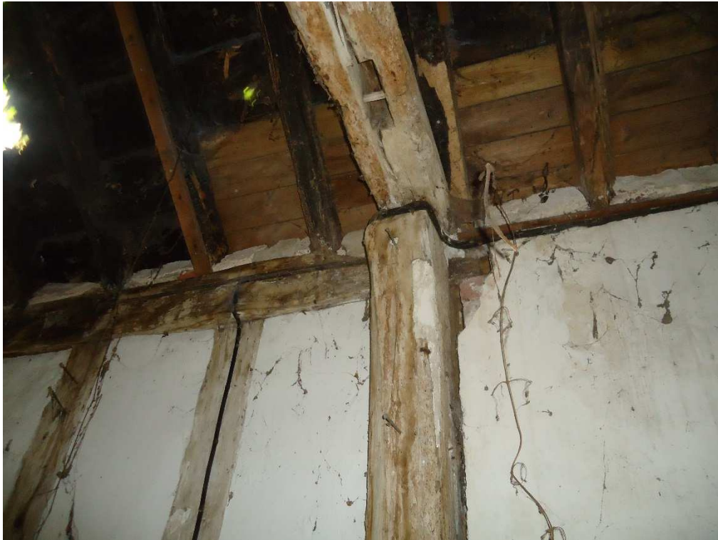
Figure 37: West end truss of the C17 structure.
