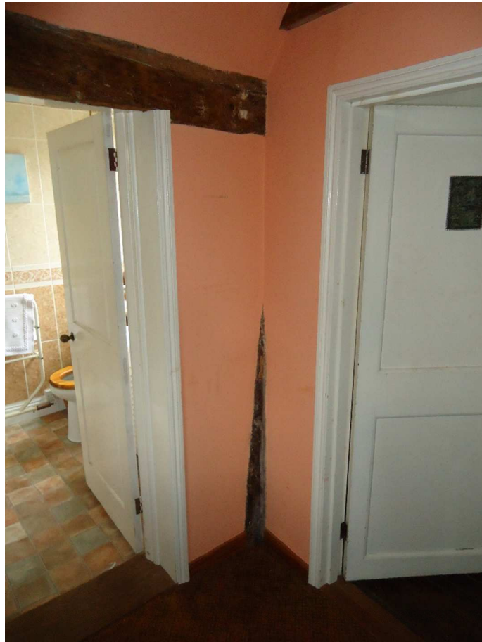
Figure 46: Ground floor - internal south elevation of the brick range.
