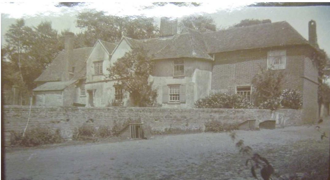
Figure 13: Rear elevation of the Pound Farmhouse.
