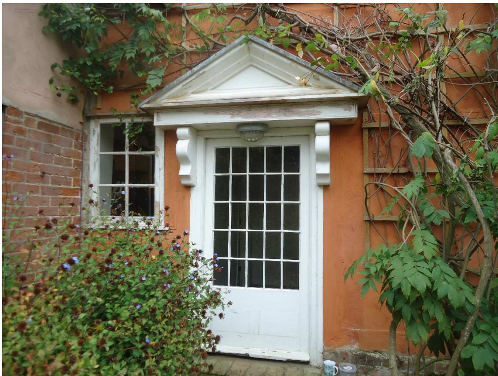
Figure 48: View of the 20 th century back door and window.
