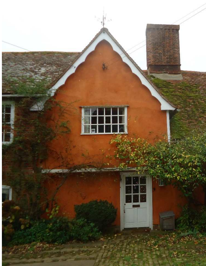
Figure 23: Early C17 jettied cross wing to south of the hall.
