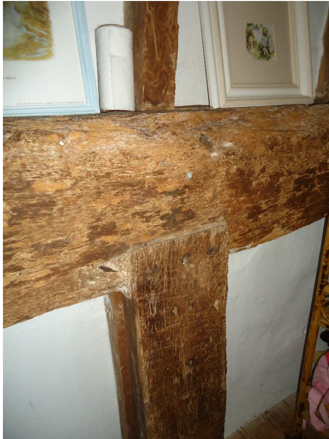
Figure 33: Inserted post underneath Truss 2.
