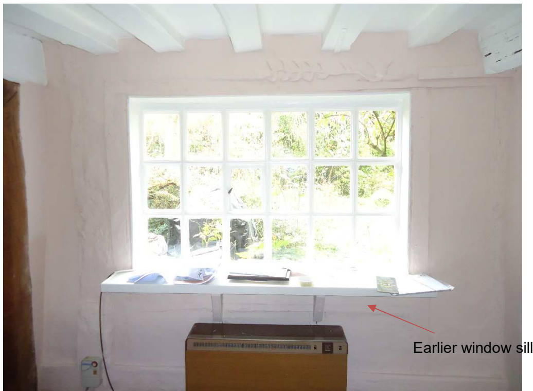
Figure 22: Evidence for a window in the high end of the hall.
