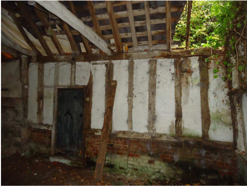
Figure 39: Doorway into lean-to structure formerly attached to the north elevation.
