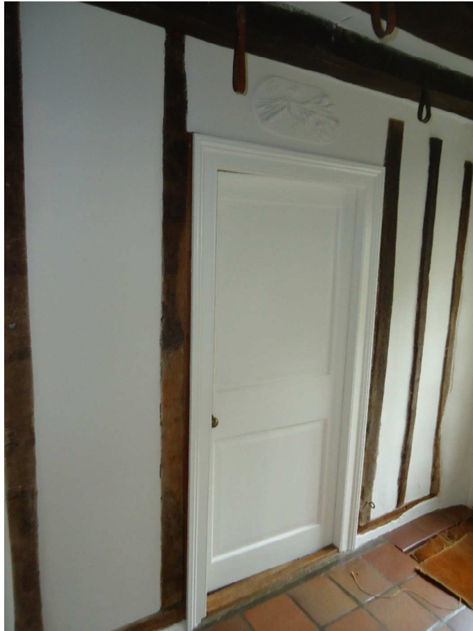
Figure 21: Inserted C18 partition wall into low end of the hall.
