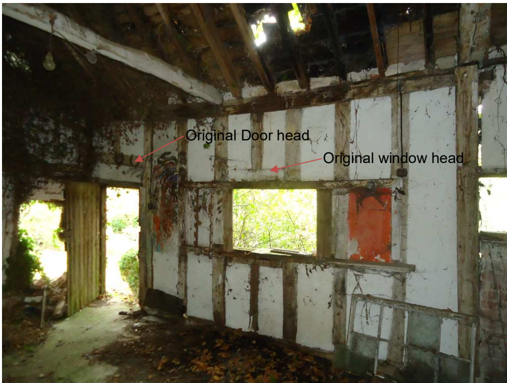
Figure 36: Internal view showing location of original door and window heads.
