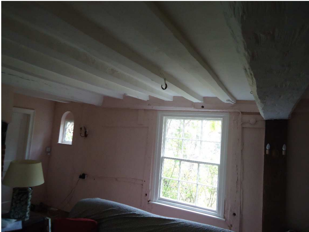
Figure 19: Inserted C17 floor structure over the hall.
