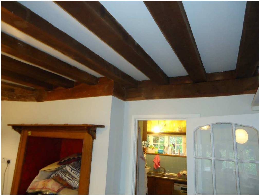
Figure 49: Inserted 20 th century kitchen fireplace and joists.
