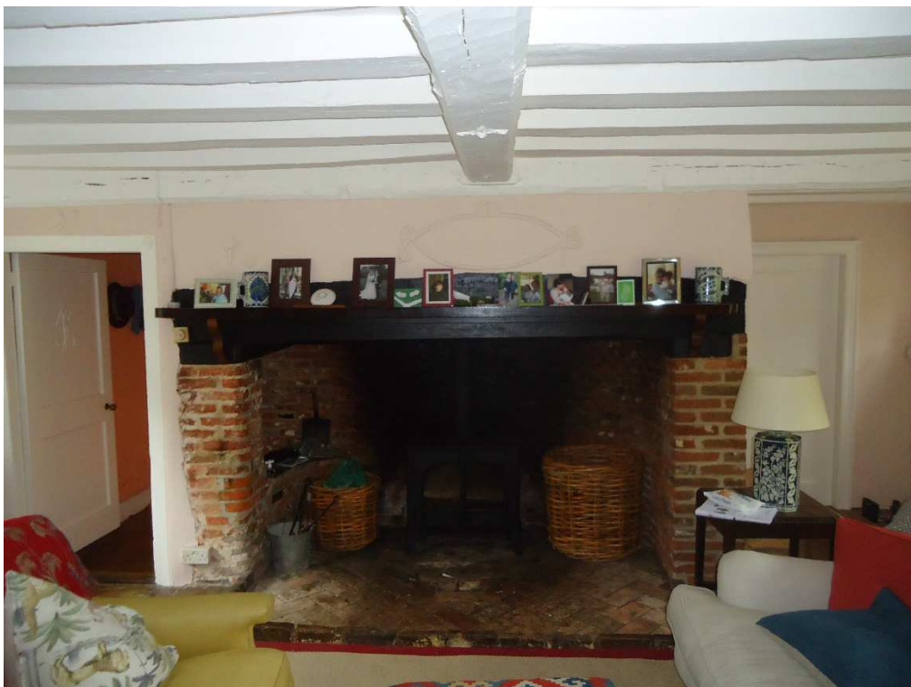
Figure 24: Inserted C17 inglenook fireplace in the hall.
