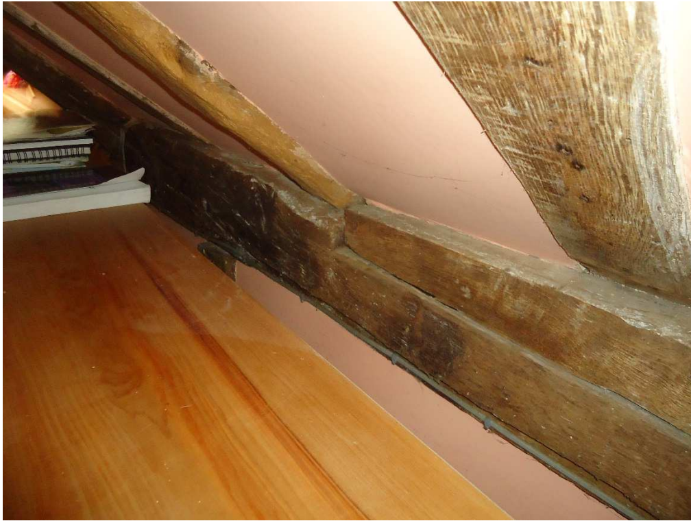
Figure 27: C17 scarf joint in front wallplate.
