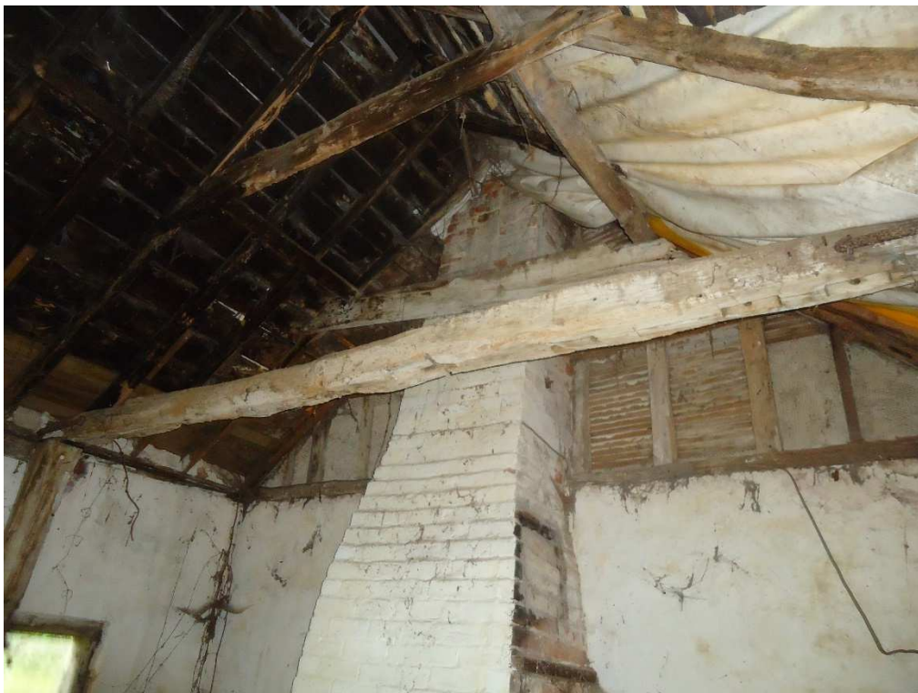
Figure 38: C19 extension to west end of the outbuilding.
