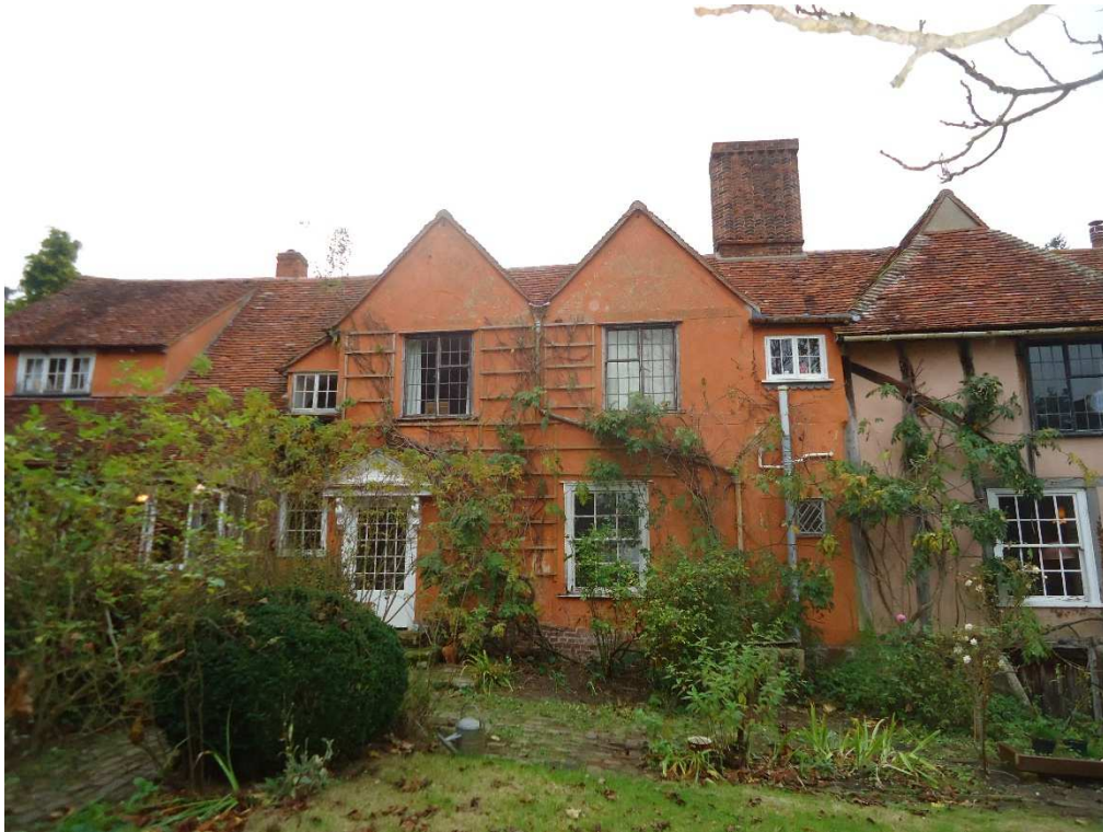
Figure 47: Double piled gable dormers to the rear of the house.
