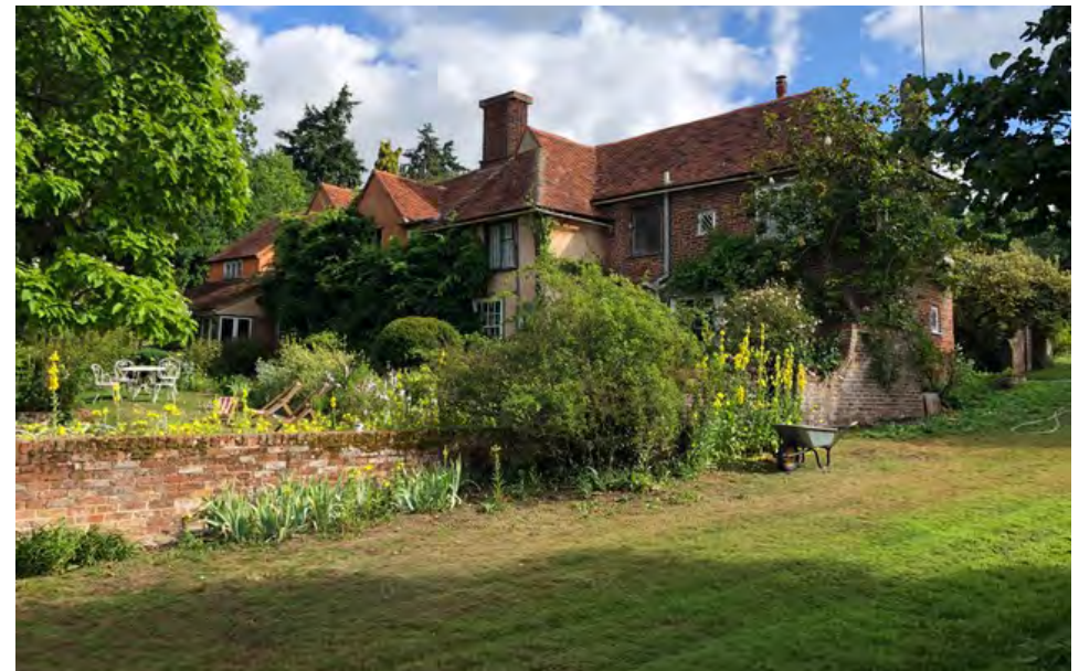
South west elevation, showing 18/19th century brick range, 17th century cross wing, and 20th century alterations to the 16th century wing beyond
