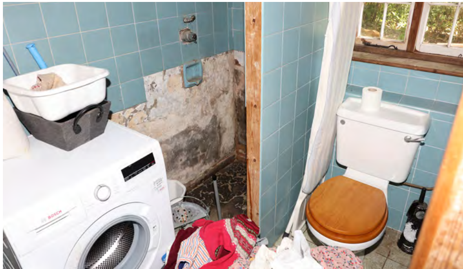
Future Back Hall to be formed by removing 20th century partitions
