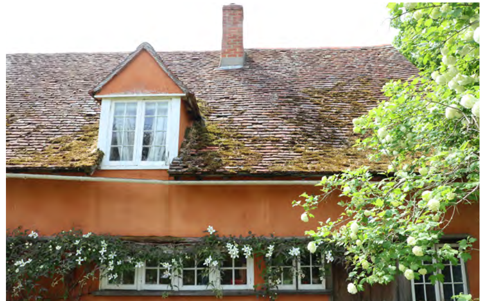
20th C dormer window in Bedroom 2, introduced when the room was changed to a bedroom. Similar dormer proposed to the current playroom between the rafters to provide light to an otherwise underlit room.
