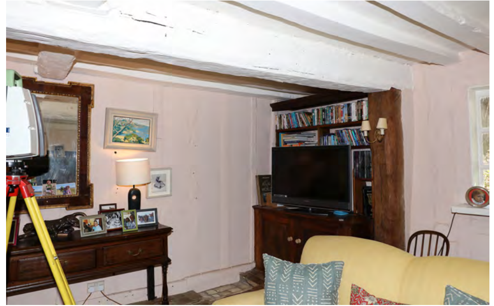
Location of proposed reopened doorway - one 20th century sawn softwood stud to be removed (see step in floor)
