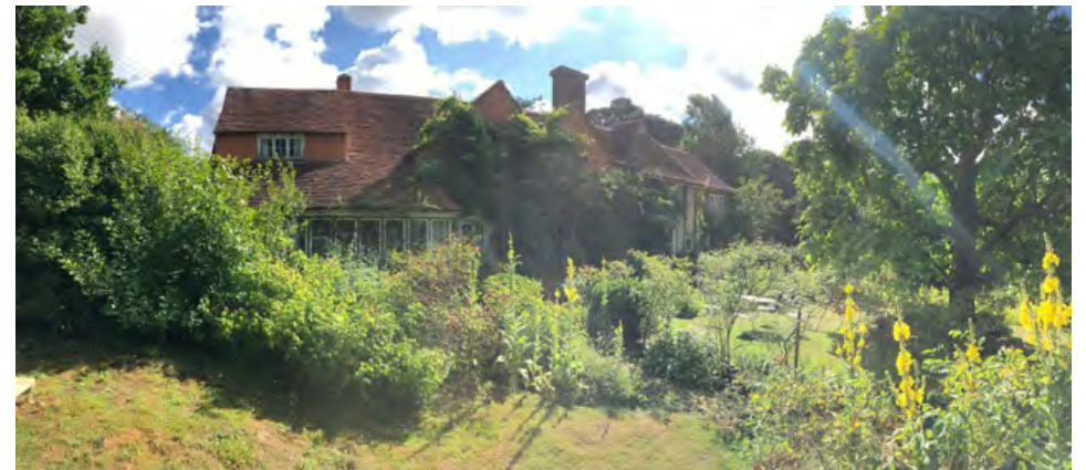
View of 20th century alterations to 16th century kitchen range
