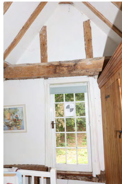
Left: 20th C Bedroom 2 dormer - between rafters - in modern plasterboard
