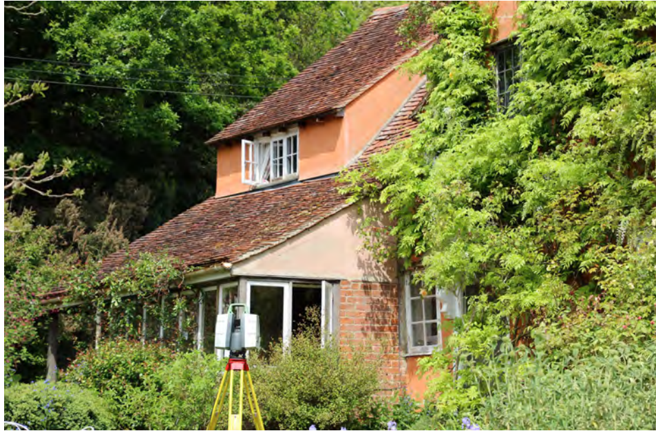
20th C dormer and bay extensions to northern service end
