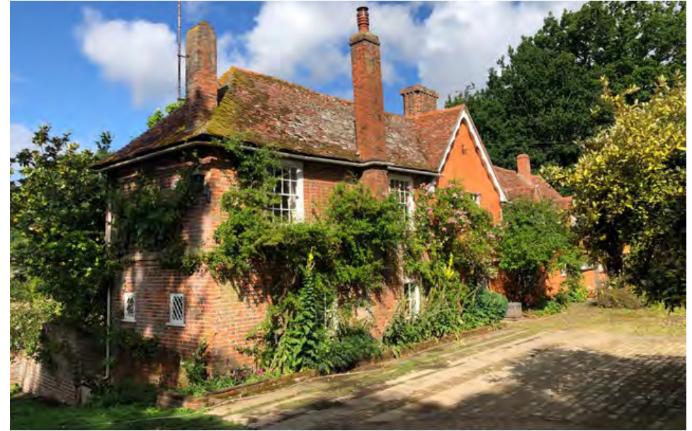
North east elevation showing late 18th/19th century brick range, and 17th century cross wing beyond
