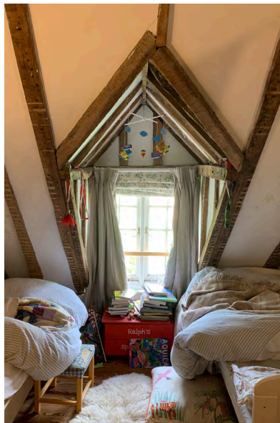
Left: 20th C Bedroom 2 dormer - between rafters - in modern plasterboard
