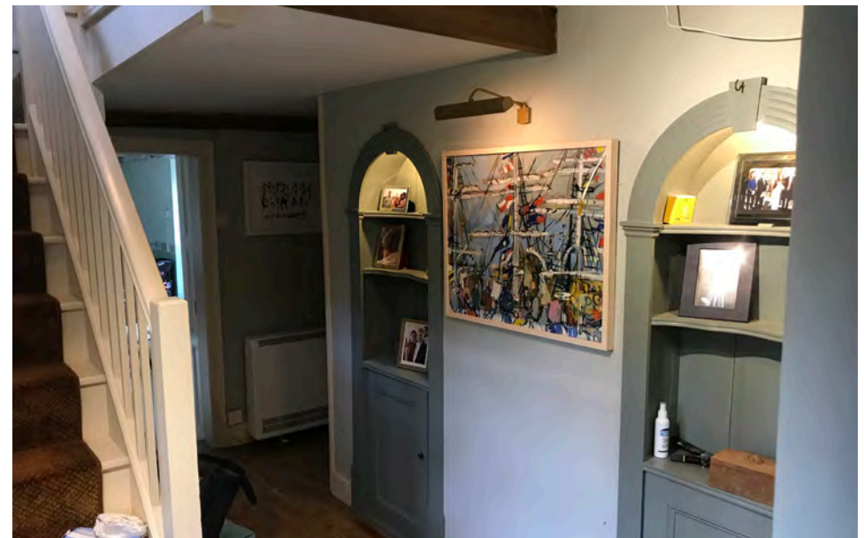
Modern stair, ceiling structure and partitions in the Entrance Hall (obstructing the view seen from Wright's painting on page 18)
