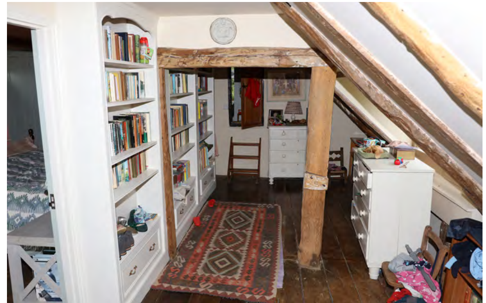
Library Corridor inserted to form central bedroom
