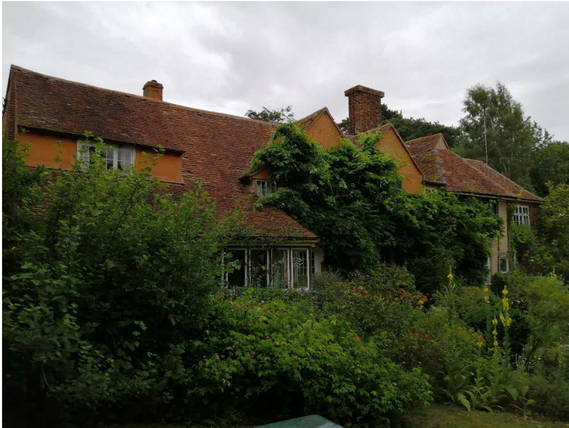
Photograph 3: South-west elevation of the house
