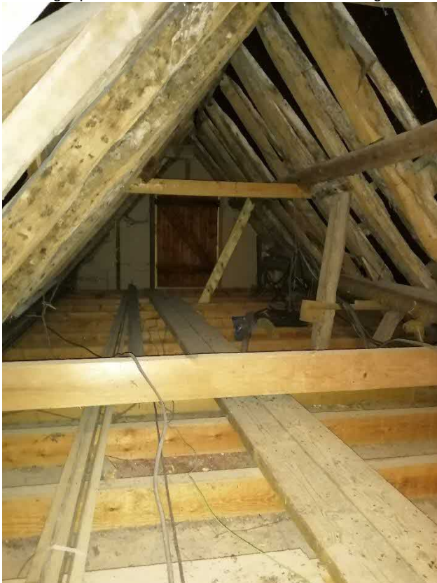
Photograph 6: House roof void (west-central)
