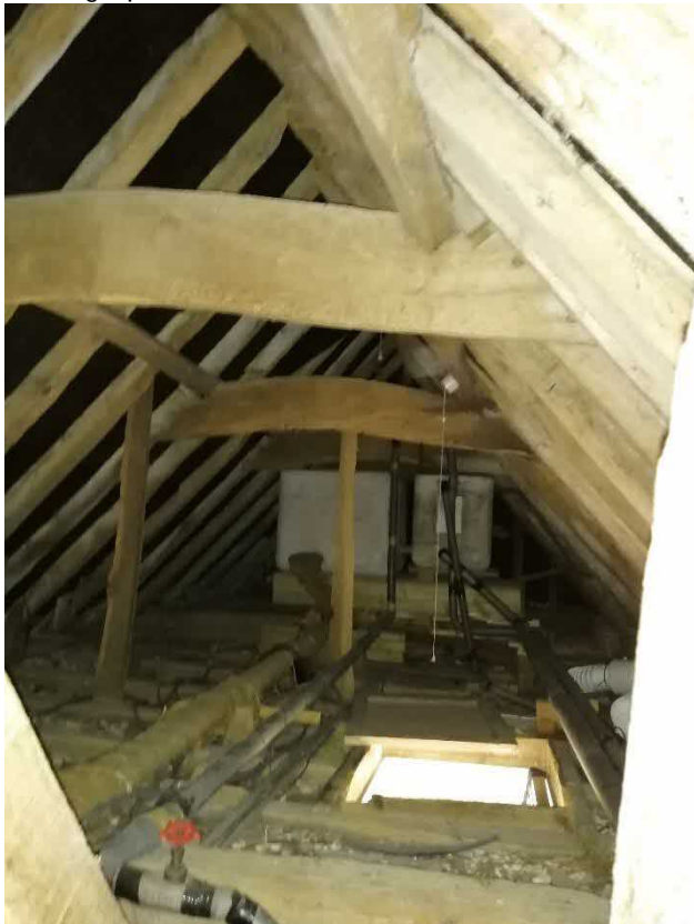
Photograph 4: House roof void (east-central)
