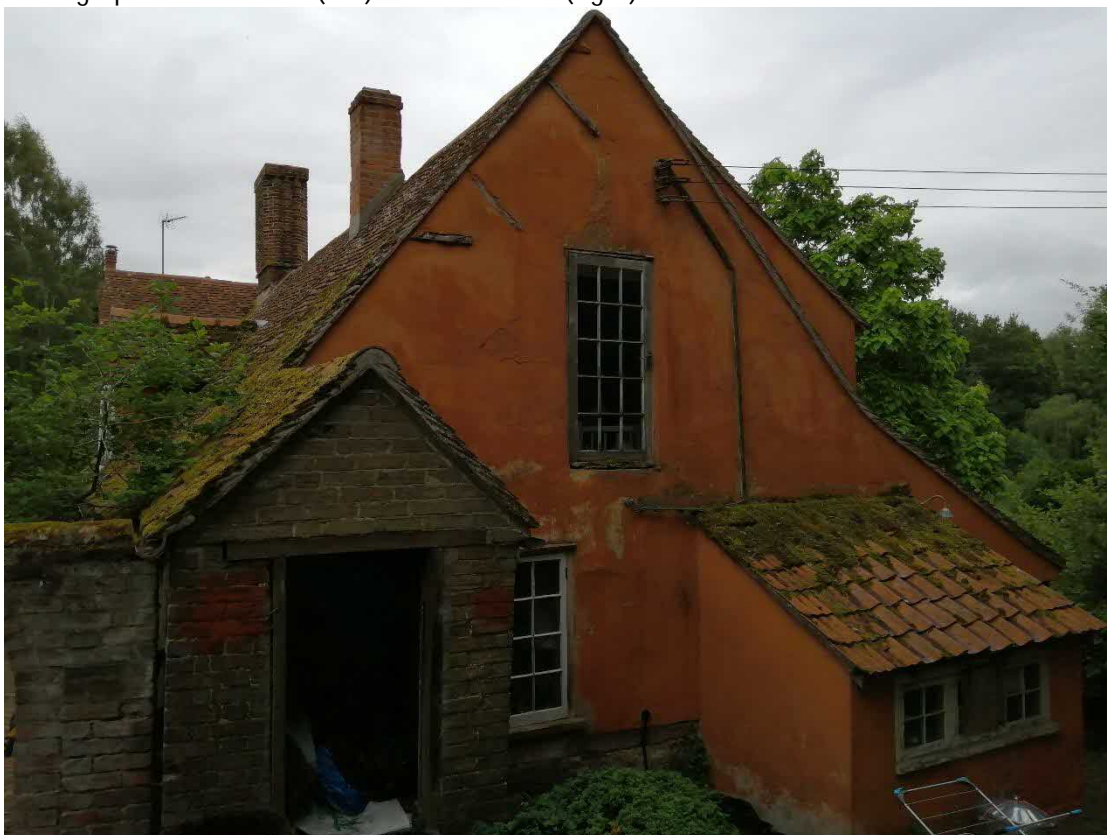
Photograph 2: North-west elevation of the house
