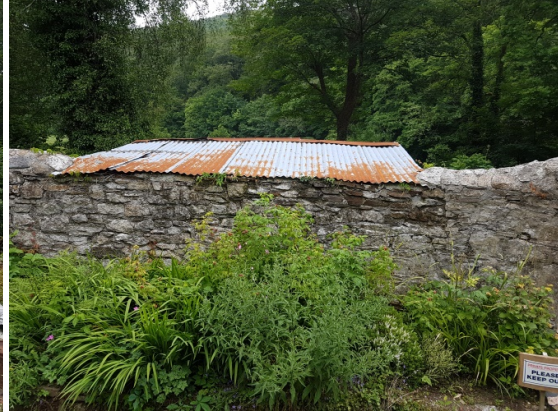
Photo 5: Rear (West) elevation.
