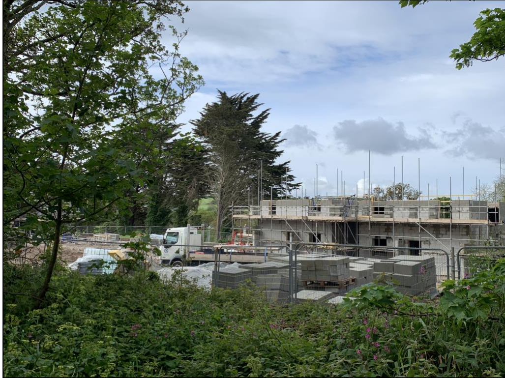
The view looking east towards the front elevations of Plots 17, 18 and 19
