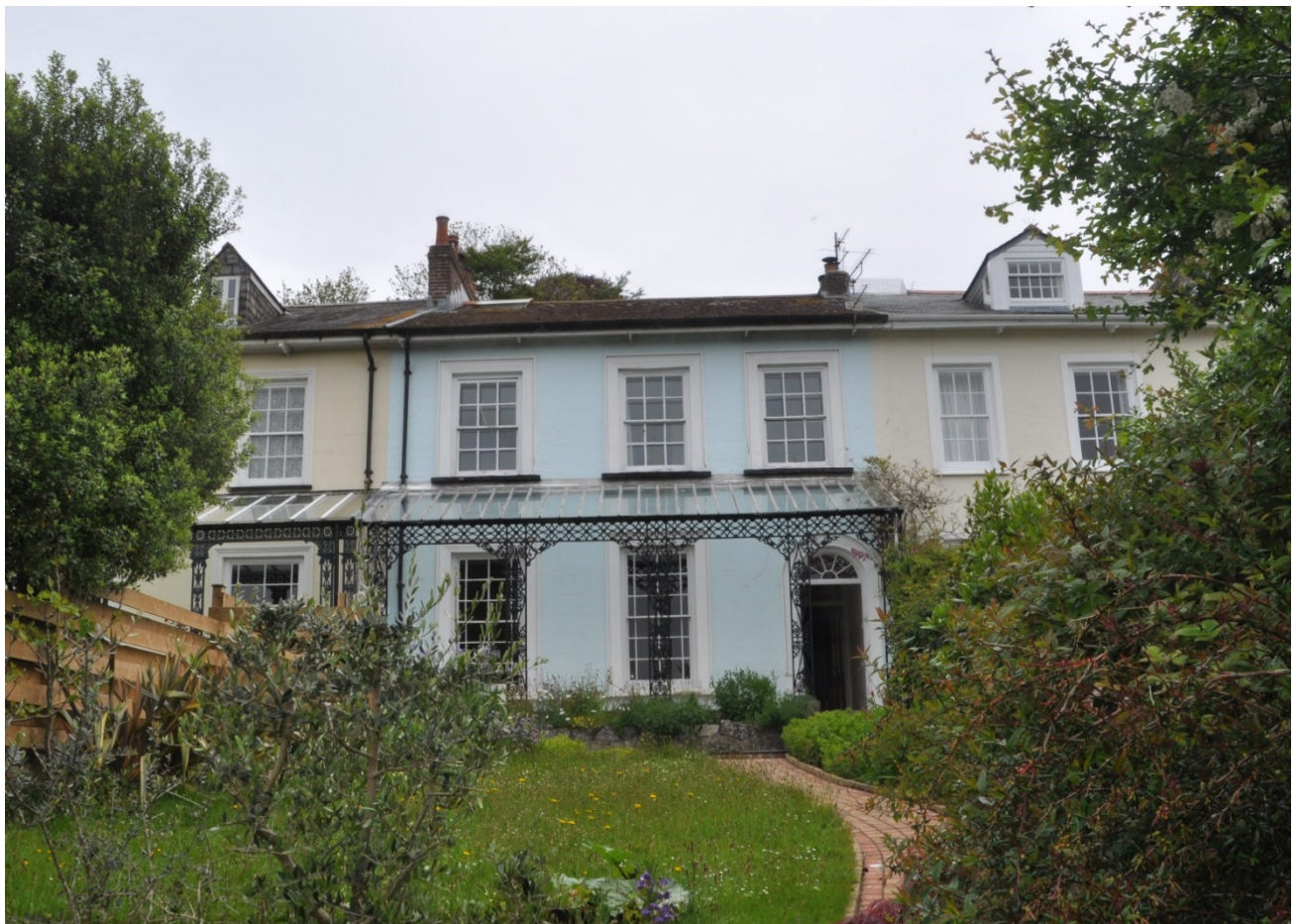
Fig 1: View of existing front elevation
