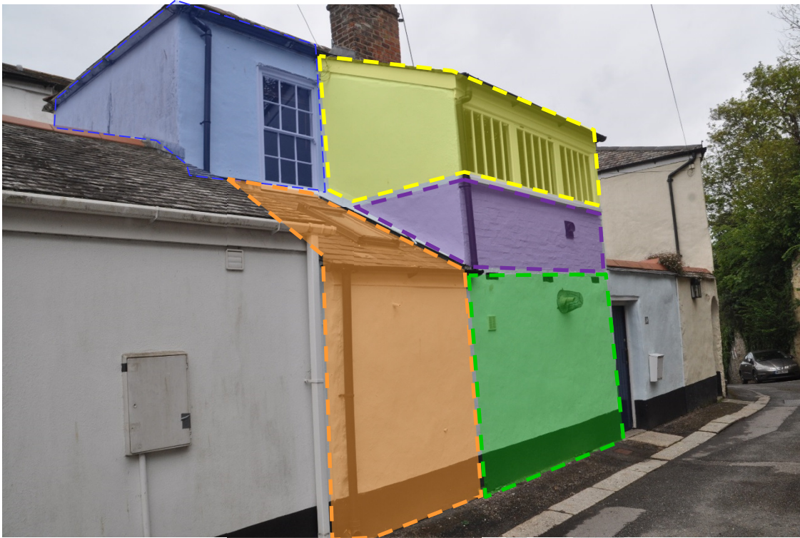
Fig 5: Existing building as viewed from rear access point.
