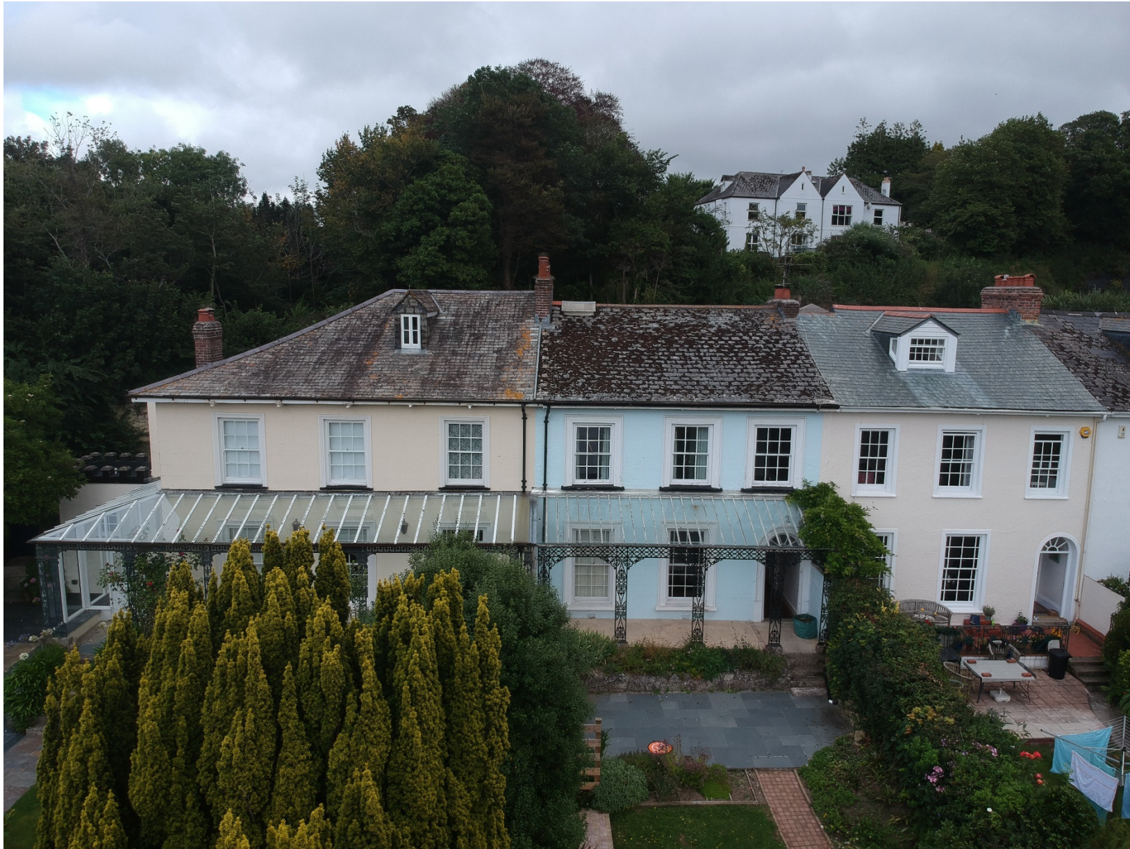
Fig 20: Drone imagery from front of site.
