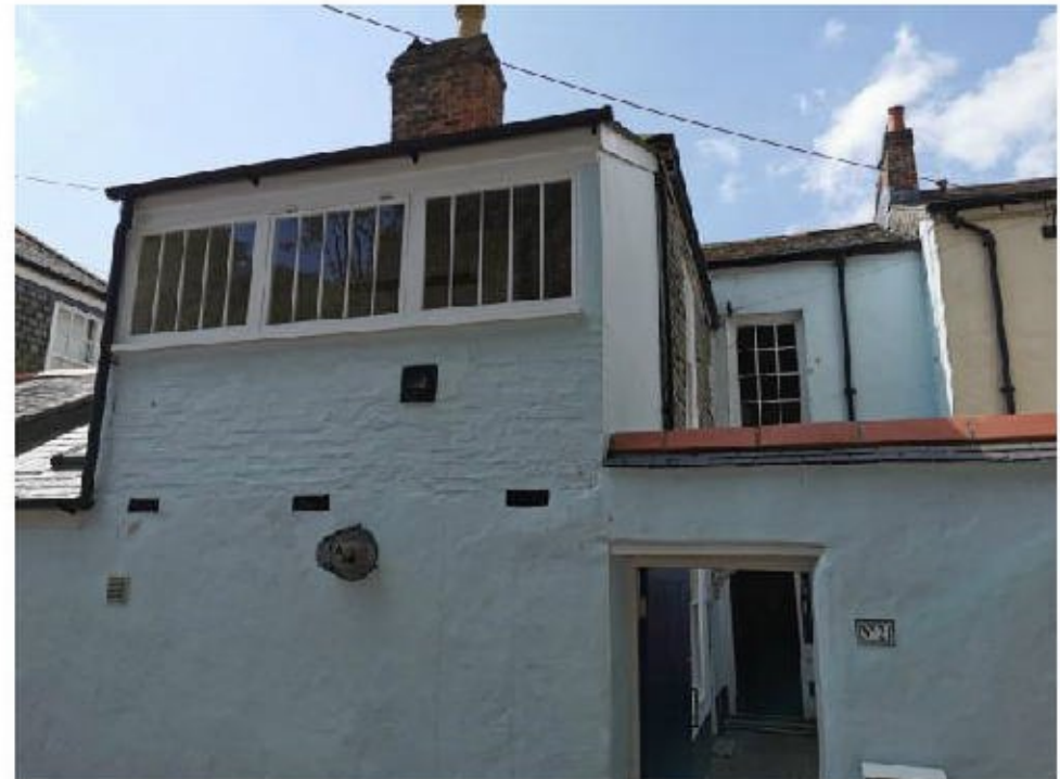
Photo 2. Showing the eastern side of the house including the extension
