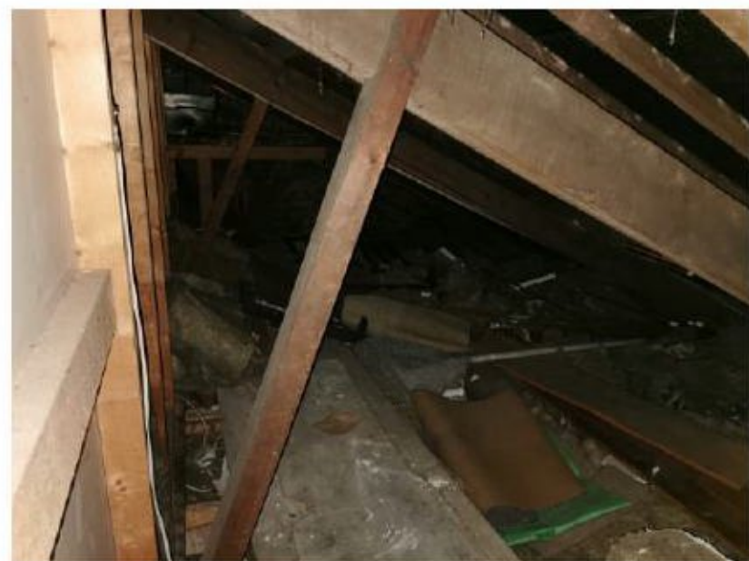
Photo 6. Showing the remaining area of roof void to the east
