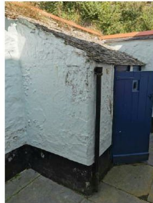
Photo 4. Showing the outbuilding
