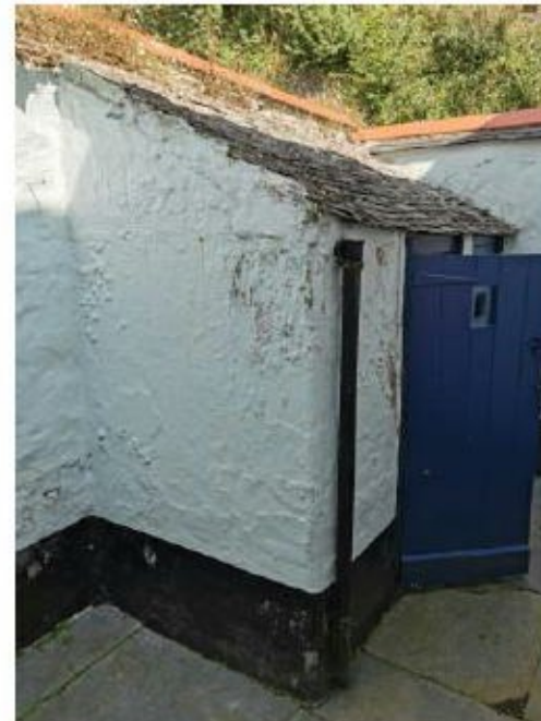
Photo 4. Showing the outbuilding
