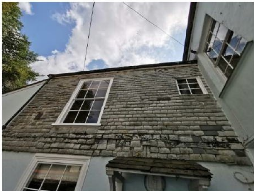
Photo 3. Showing the wall hanging slates on the rear extension
