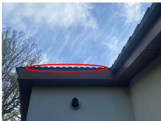
Plate 11: Access points at edge of roofline
