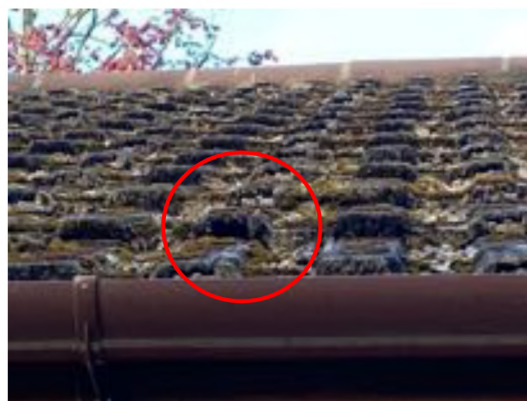
Plate 8: Access point under tiles
