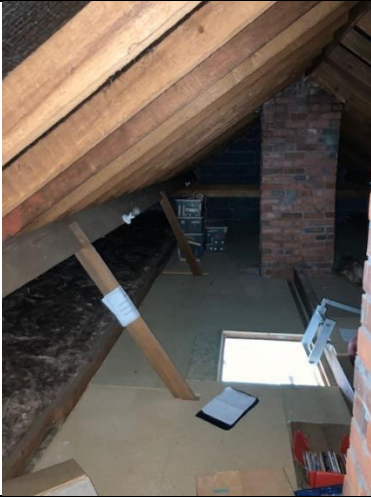
A.7 Main loft above two storey section
