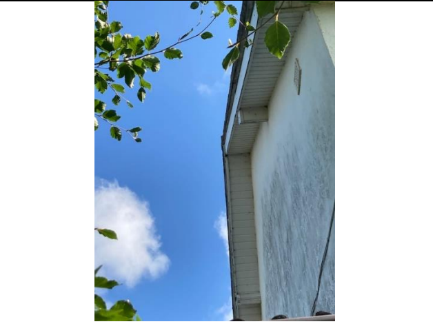
A.4 Sealed soffit on eastern gable
