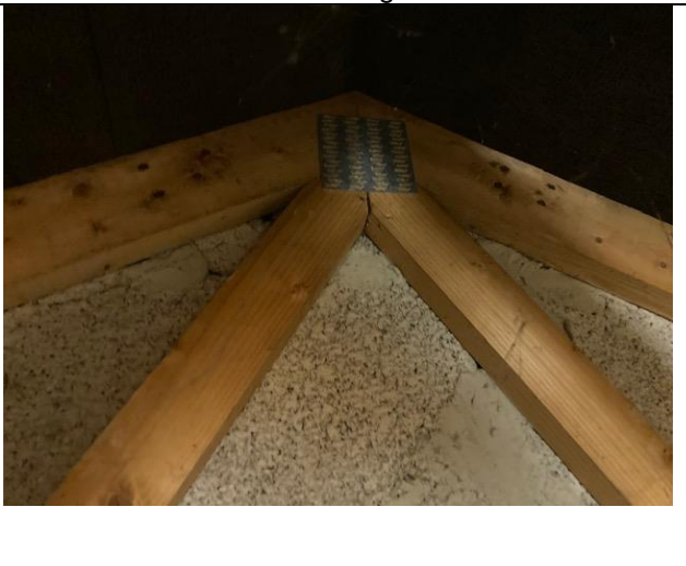
A.6 Sealed end rafter in extension loft
