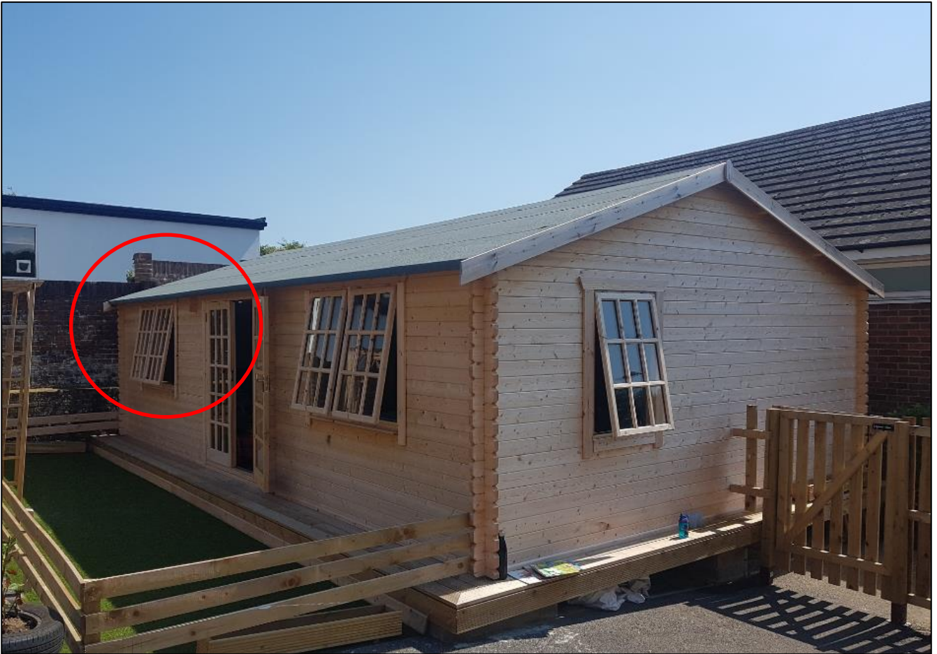
Red circle indicates where existing cabin sits entirely behind existing brickwork wall along south-eastern boundary of application site.
