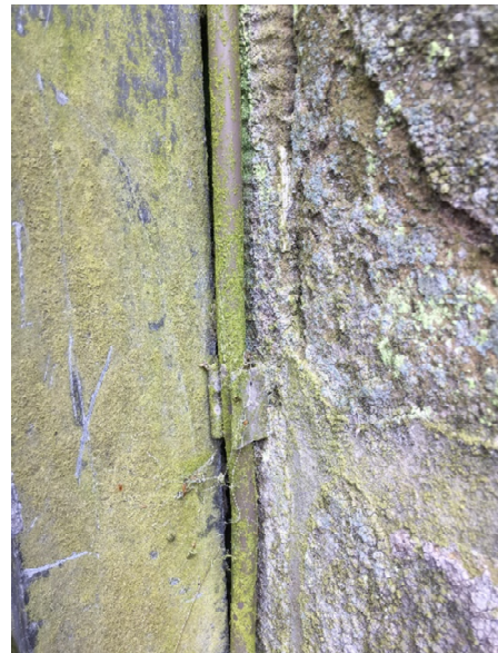
Existing Lightning Protection Fixing
