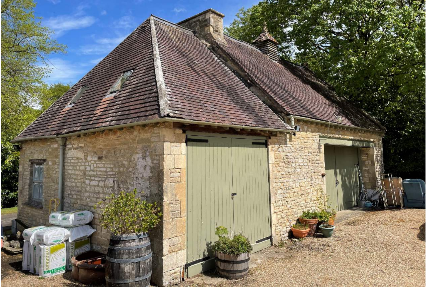
Plate 20: Coach house, south and west elevations.
