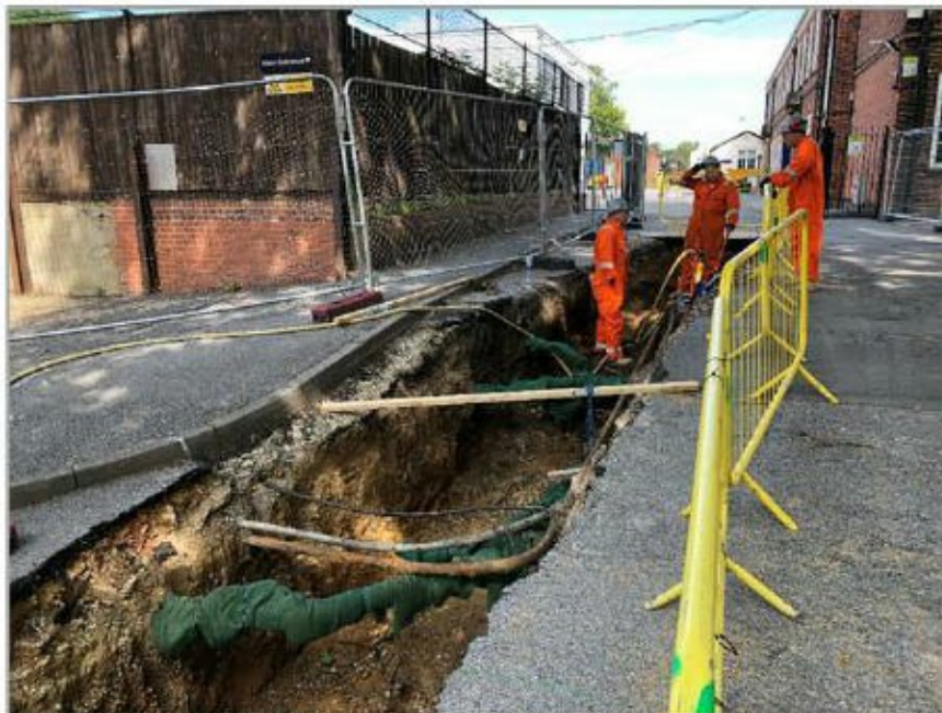
Figure 3 – Example of Retained roots in service trench
