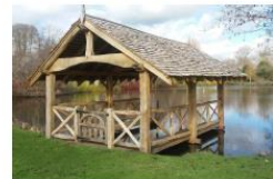
BOAT HOUSE Example of oak framed boat house with shingles to roof
