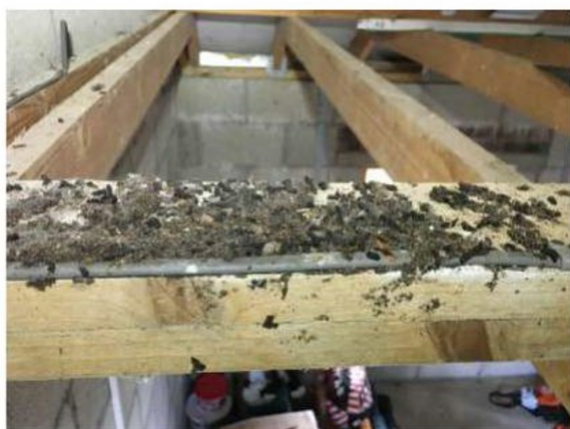
Photograph 3. Bat droppings on central beam.
