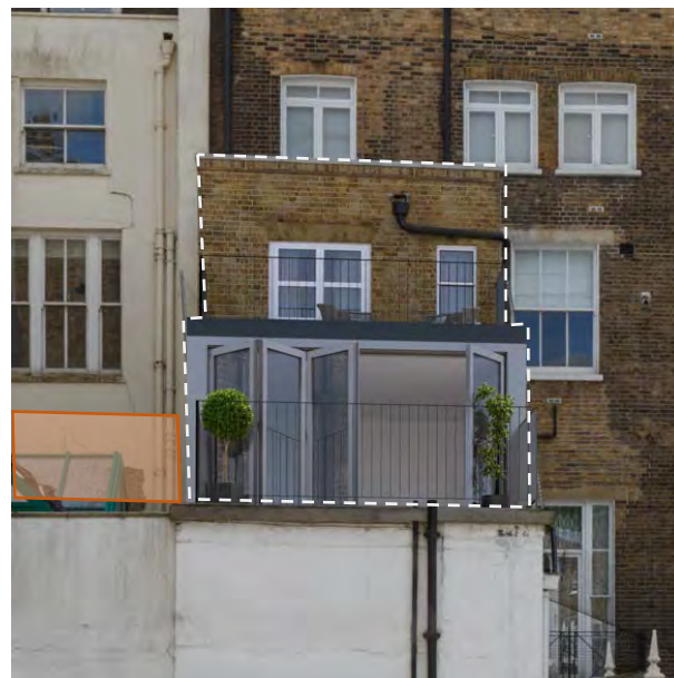
Figure 29 and 30: As existing and as proposed image of proposals from the rear. Hatched orange, a scheme consented in 2018 shows additional height approved at number 2. A new submission has been made for this site since so it remains unclear what the ultimate ambition of the applicant is for the site.
