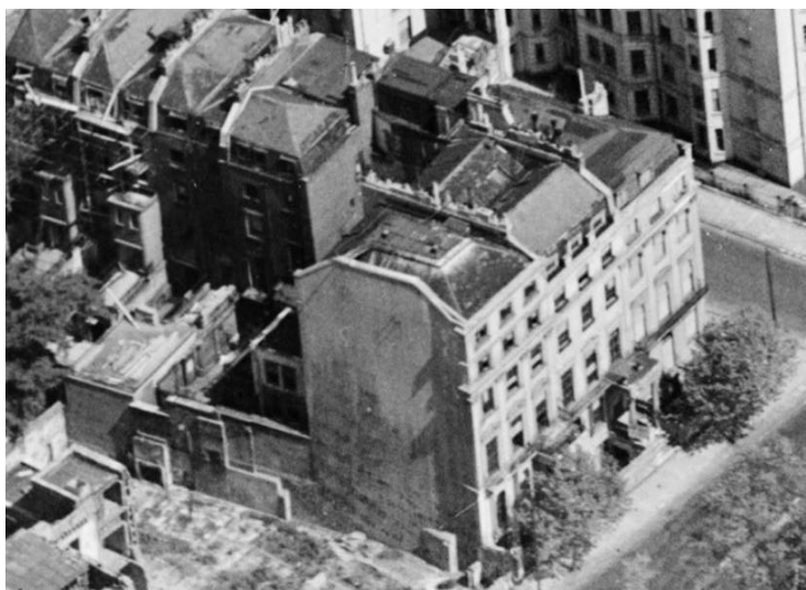
Figure 11: Aerial images from 1946 indicating the complete removal of the adjoining No.4 Hyde Park Place. The subject rear closet wing of No.3 Hyde Park Place can be seen in this image (c. Britain From Above)
