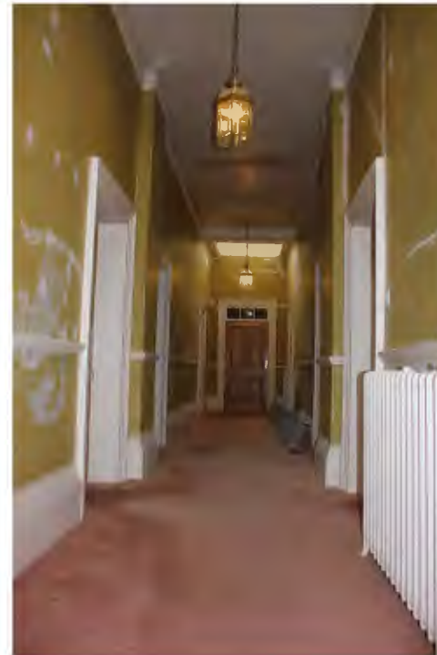
First floor bedroom corridor
