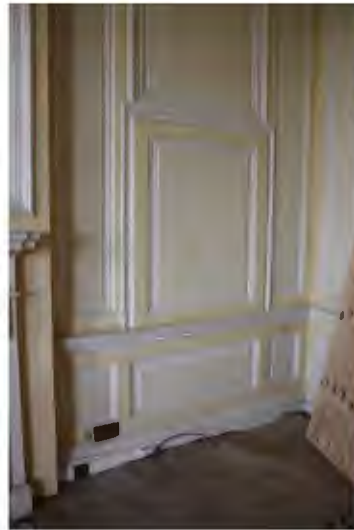
Blocked jib door in the Drawing Room, looking west.
