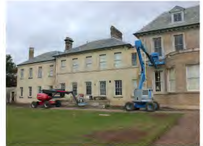
South elevation, west wing
