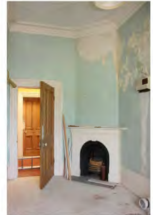
Former dressing room with corner fireplace
