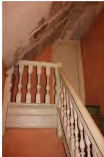
Back staircase from phase one with entrance to attics
