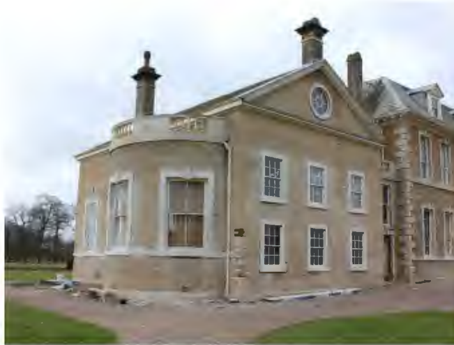
Pavilion northern elevation and bay window
