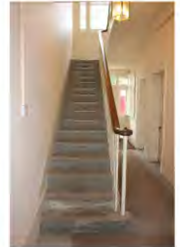
Open string stone back staircase
