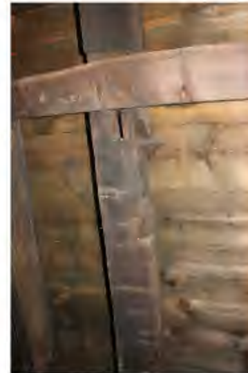
Evidence of reused timbers
