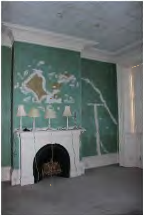
Bedroom FF12 with decorative cornice, marble fireplace and cast-iron grate and window shutters
