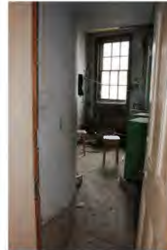
Former bakehouse (now boiler house with original floor, window, and rising shutter
