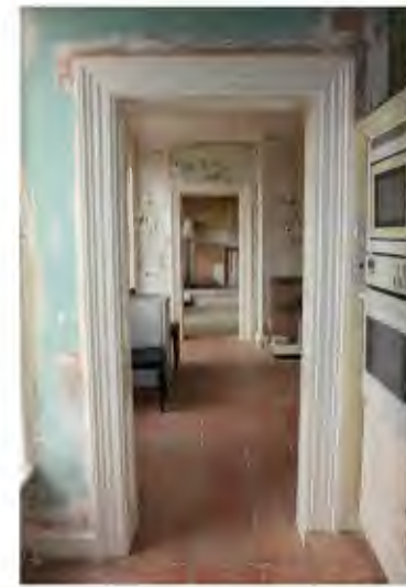
Inserted doors through GF12 to GF13. Note the foreground space was formerly a Victorian WC
