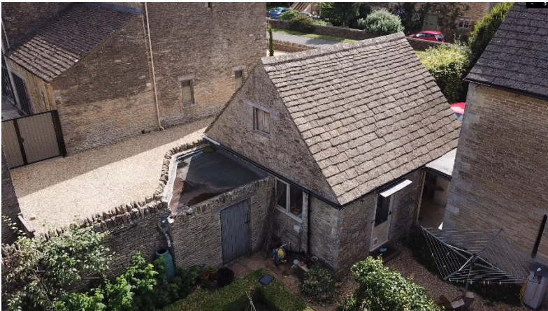
Existing rear of garage showing existing store that is to be removed.
