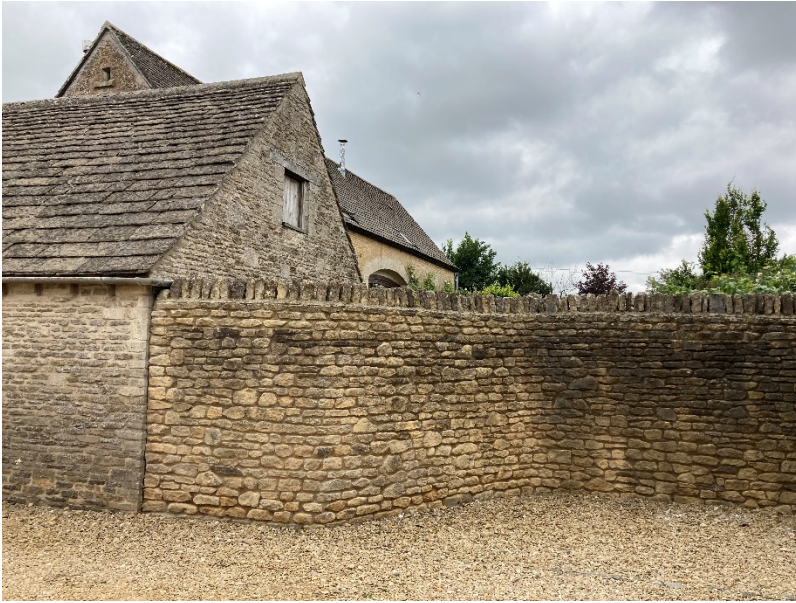
View of existing boundary wall and garage taken from Grange Barn. Photograph showing existing cock and hen capping proposed to be removed to allow installation of a lead flashing.
