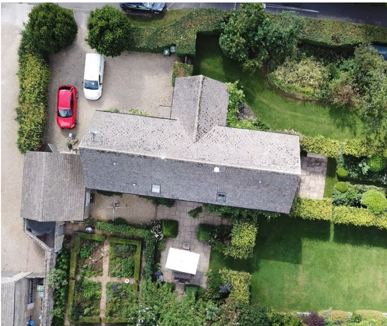
Aerial view showing existing parking arrangement.
