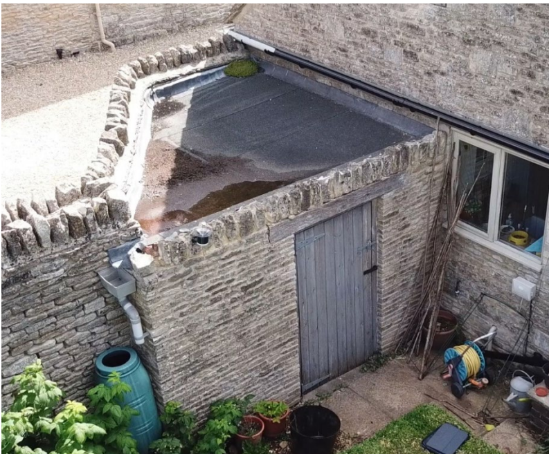
Existing store with flat roof and lead flashing into boundary wall.
