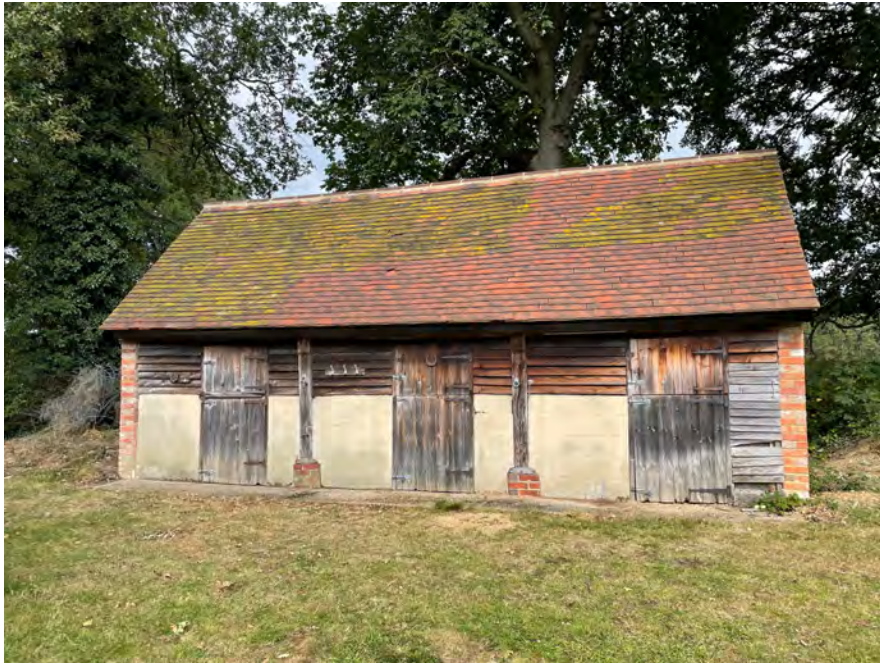
View of stables
