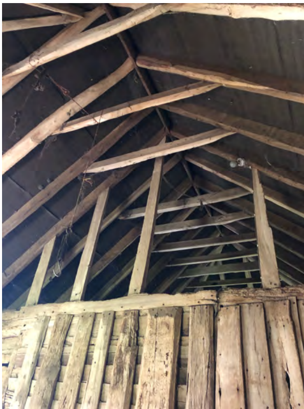
Barn interior – roof structure
