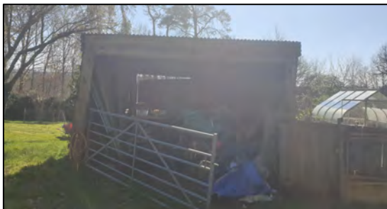
Photograph 5: Building B4. Photograph taken by Tara Hall on 25 th March 2020.
