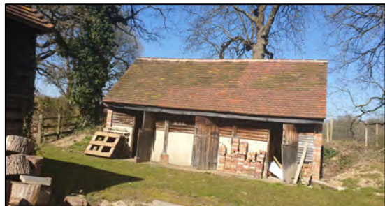
Photograph 6: Building B2. Photograph taken by Tara Hall on 25 th March 2020.
