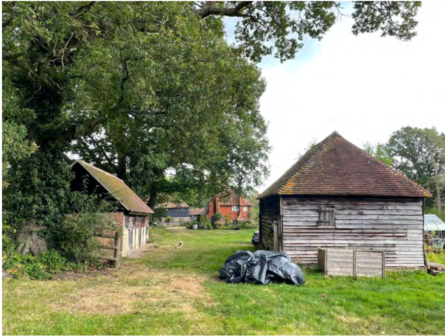
View of west end of barn and stables
