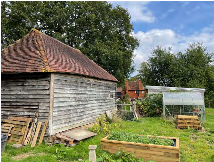
View of south west corner of barn and woodshed
