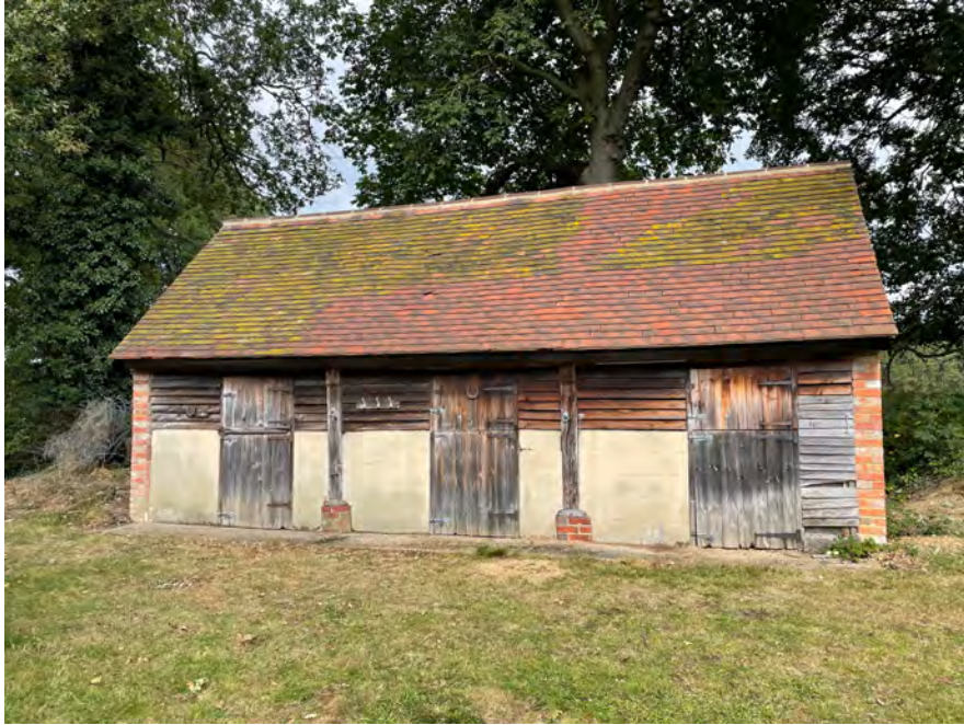
View of stables
