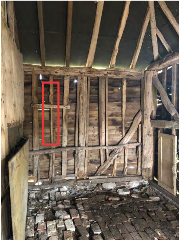
Barn interior – south elevation red box indicates area of new window
