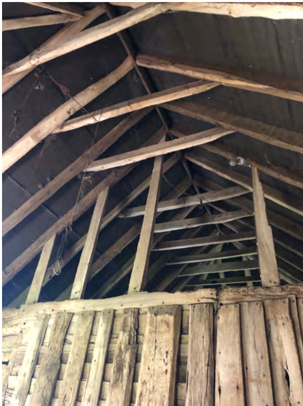
Barn interior – roof structure
