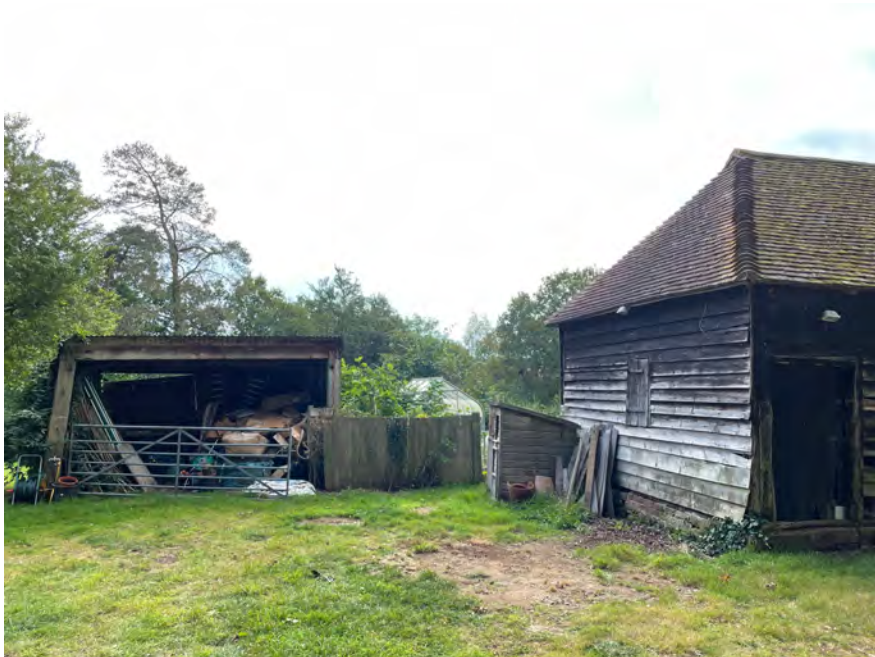
View of east end of barn and woodshed
