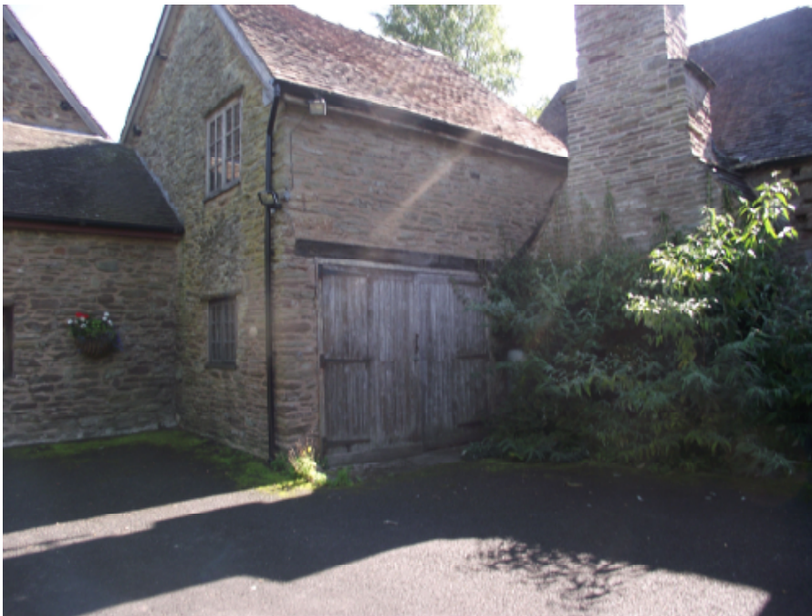
Garage doors to be replaced.
