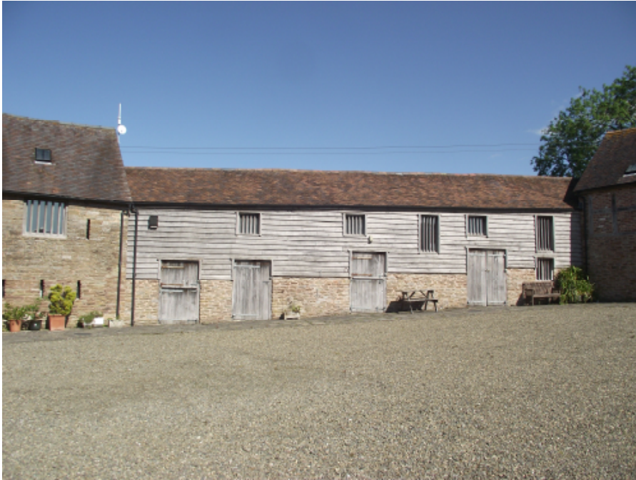
External view of barn 2.
