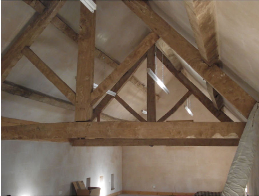
Internal image of trusses in first floor of barn 1.
