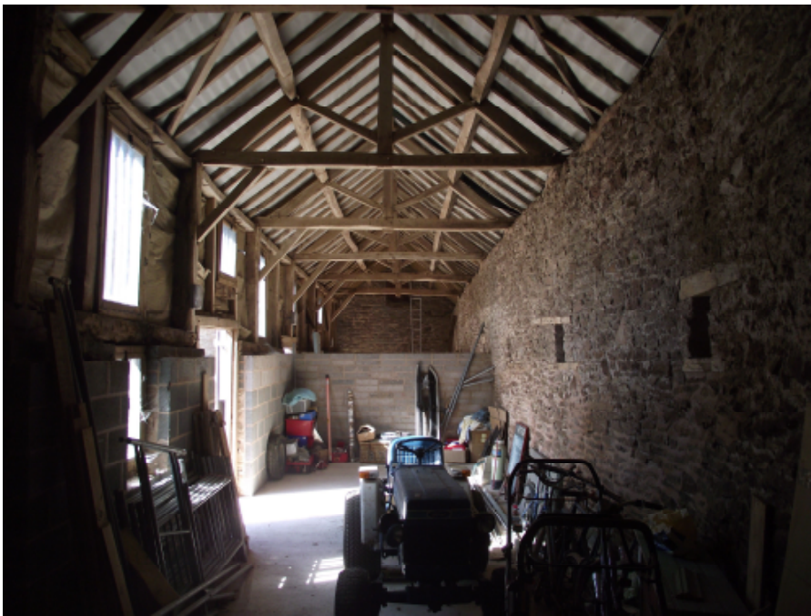
Internal view of barn 2.
