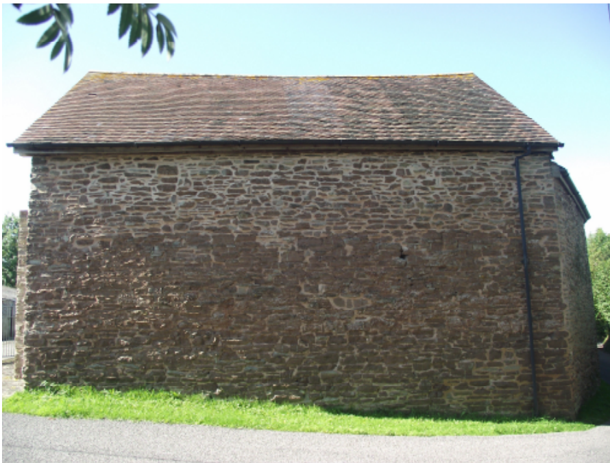
East road elevation of annex.
