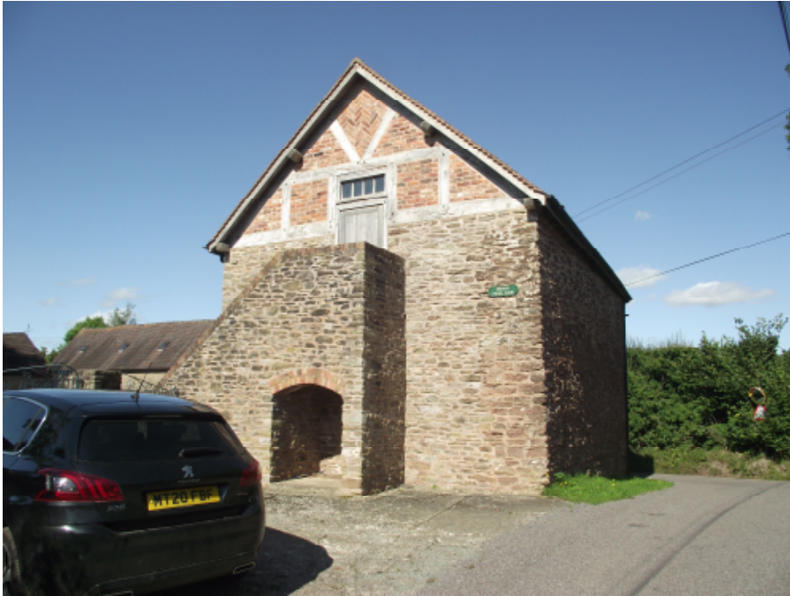
South gable of annex.
